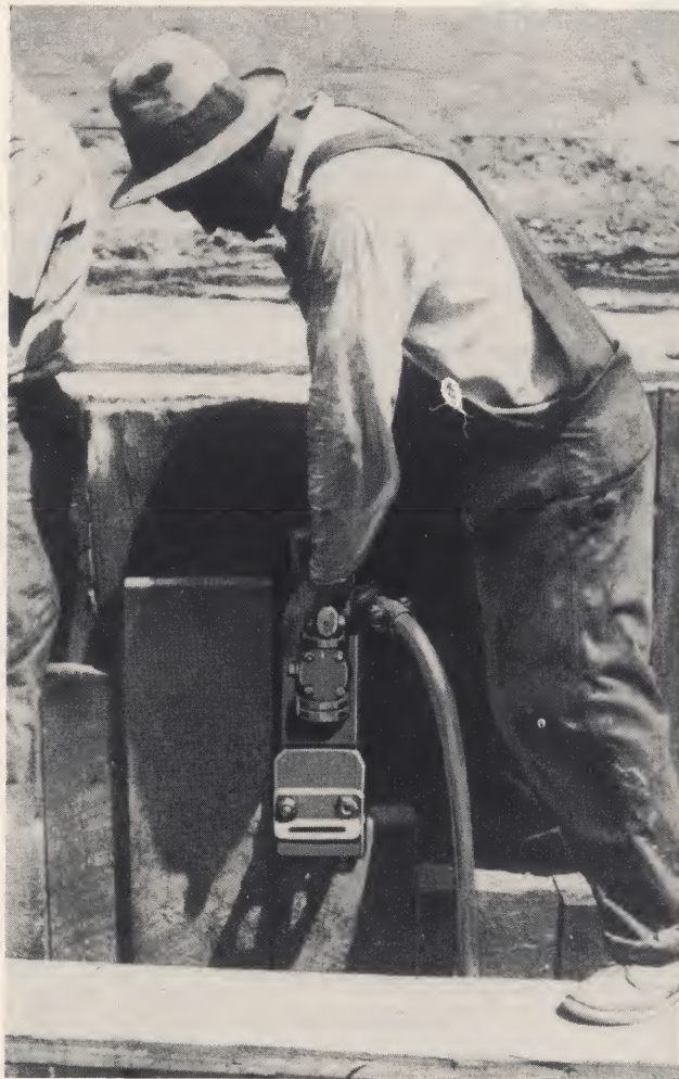
Great Neck, N. Y. McKiernan-Terry No. 0 and No. 1 Double-Acting Pile Hammers used to drive wood sheeting in laying a sewer. A total of 7,000 feet of 2-inch x 8-inch sheeting 25 to 32 feet long were driven through
