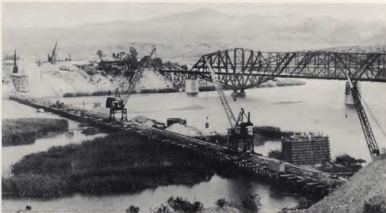
Topock, Ariz. McKiernan-Terry No. 10-B-2 Double-Acting Hammers driving semi-circular double-wall cofferdams into cemented volcanic gravel and boulders, in the construction of the Santa Fe Railroad bridge shown in foreground of upper picture. Kansas City Bridge Co., contractor.
