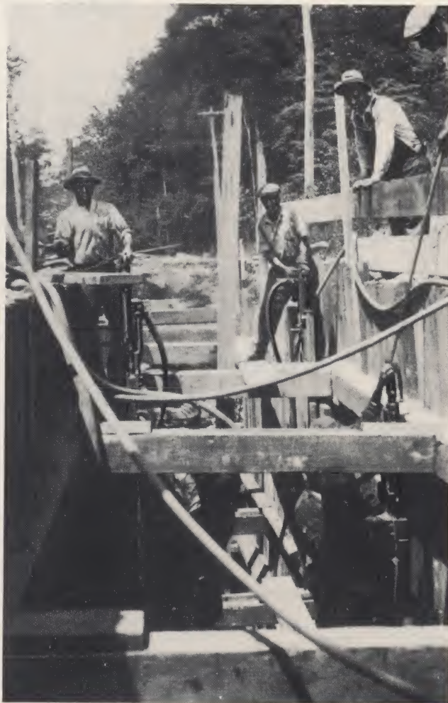
sandy loam, stone, gravel and clay mixture. The No. 0 Hammer was used to drive an average of 180 pieces 2-inch x 8-inch x 20-feet to a maximum penetration of two feet. Then No. 1 Hammers were substituted.
