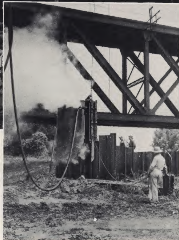
(Right) Cairo, Ill. McKiernan-Terry No. 9-B-3 Double-Acting Hammer driving steel sheeting for a 1½-mile cellular-type flood wall, to be flanked with levees. Part of the 20-mile chain of walls and levees protecting Cairo against Mississippi River floods. Project of U. S. A. Corps of Engineers. Ottinger Bros. Construction Co., contractors.
