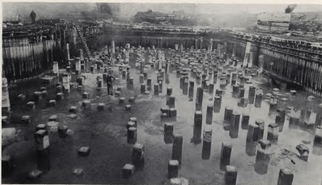
Hine, Mo. McKiernan-Terry B-type Double-Acting Hammer driving 48- to 68-foot reinforced concrete piles under water for the foundation of the Howard Bend Water Works plant for the City of St. Louis. The tops of these piles came to rest 30 feet below the surface. Other McKiernan-Terry Double-Acting Hammers, Nos. 6 and 7 were used to drive, and later pull, the steel sheet piling used for the cofferdam. Contractors, Frazier-Davis Construction Co. See also page 31.
