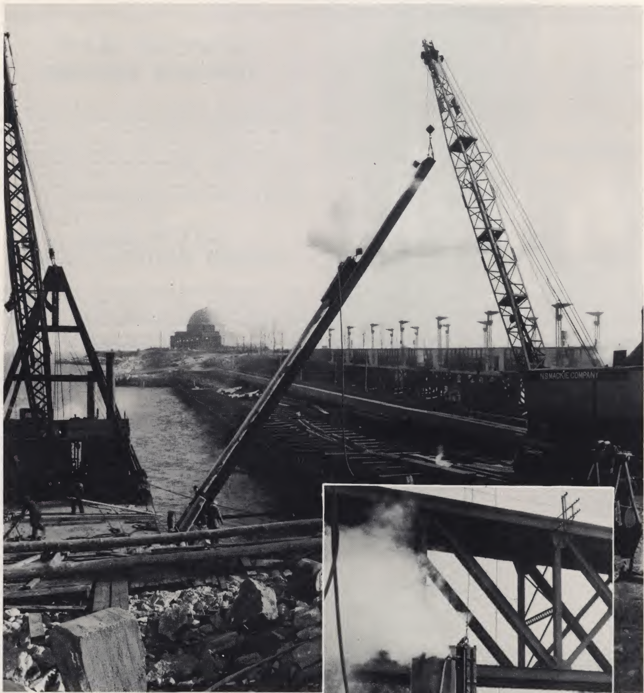
(Above) Chicago, Ill. McKiernan-Terry No. 9-B-3 Double-Acting Hammer driving batter piles for bulkheads for causeway to Northerly Island in Chicago Park District. Contractors, N. S. Mackie Co.
