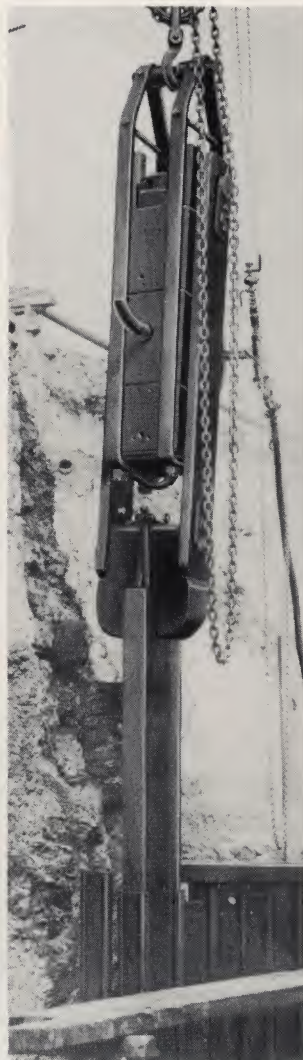
Pulling piles with inverted McKiernan-Terry Double-Acting Pile Hammers. Left —No. 6 Hammer pulling 14-inch arch web steel piling, using standard rig shown at right of page. Center —Pulling sheet piling 44 feet long, concreted to a depth of 41 feet—without difficulty. Right —Special pulling rig, used in England, made of steel bars with grips to pile webs.
