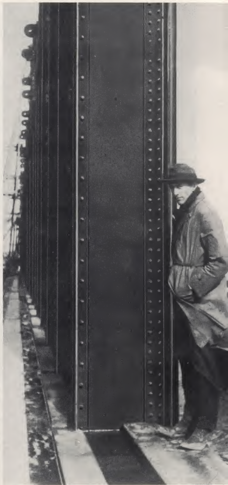
Jacksonville, Fla. McKiernan-Terry No. 11-B-3 Double-Acting Hammer driving steel sheet piles for the municipal dock on the St. John's River. The job required 3600 lineal feet of 12-inch piling, with every 6 sheet piles separated by immense master pile. The 45-foot sheeting was driven to about 42 feet penetration through sand, mud, clay, phosphate, etc. The master piles, 55 feet long, were driven to about 52 feet penetration. Contractor, C. E. Hillyer.
