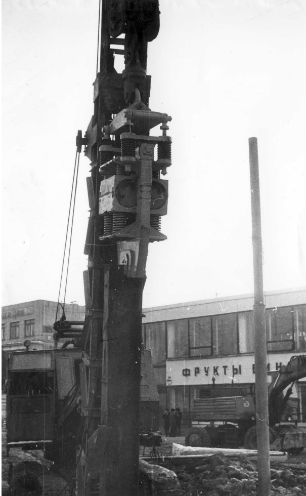
Figure 22. SP-83 Sheet Pile Extractor (from Warrington and Erofeev (1995))
