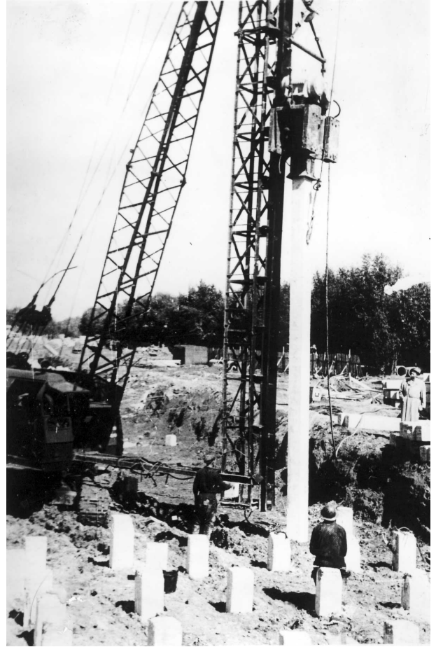
Figure 8. S-836 Impact-Vibration Hammer (from Warrington and Erofeev (1995))
