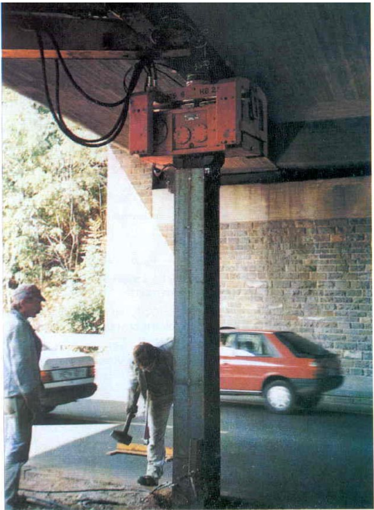
Figure 10.2-4: If the soil conditions allow the use of vibrators fixed directly to the boom of an excavator this may be a reasonable solution, as shown in the picture.
