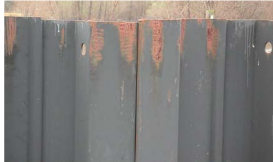
Figure 57. A relatively newly installed PZ 22 steel sheet pile showing onset of rusting
