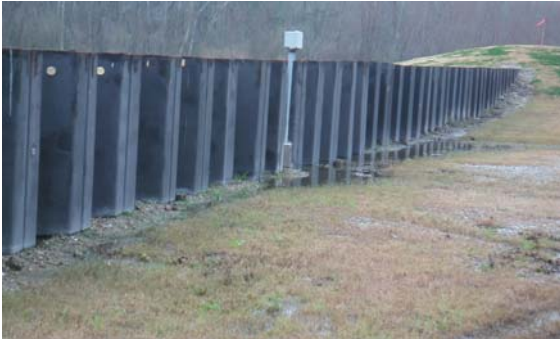
Figure 57. A relatively newly installed PZ 22 steel sheet pile showing onset of rusting
