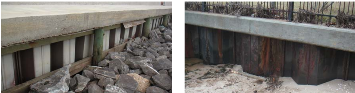
Figure 56. Clear superiority of PVC over steel for durability. Both were installed six years ago at 228 Esquinance Street, Mandeville, LA. The steel sheet piles on the right show advanced corrosion.
