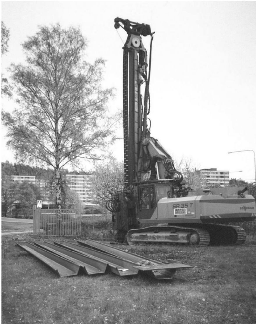
Figure 4-5 Picture taken at the Vårby test site, where the vibratory system and the sheet piles were used.
