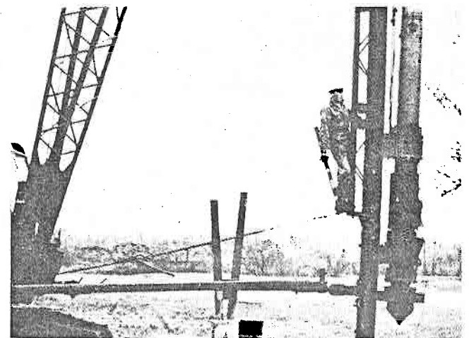
Figure 5.2. Diesel hammer.
