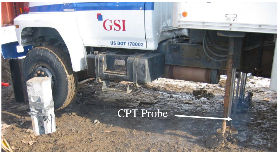
Figure 5.2. View of CPT2 test in progress, located 9 ft (2.7 m) south of UHPC pile P2
