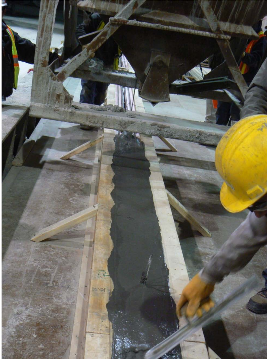
Figure 4.19. Pouring of 35-ft (10.7-m) long UHPC pile P1
