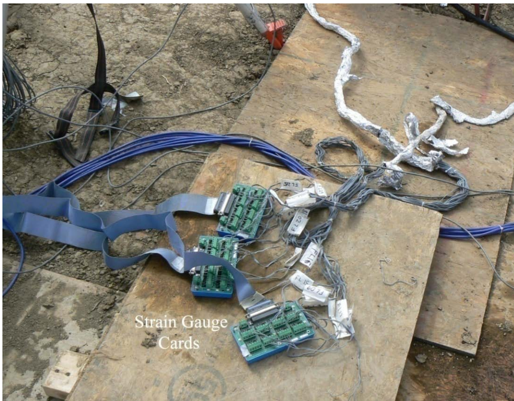
Figure 5.32. Data collection system used during the lateral load test
