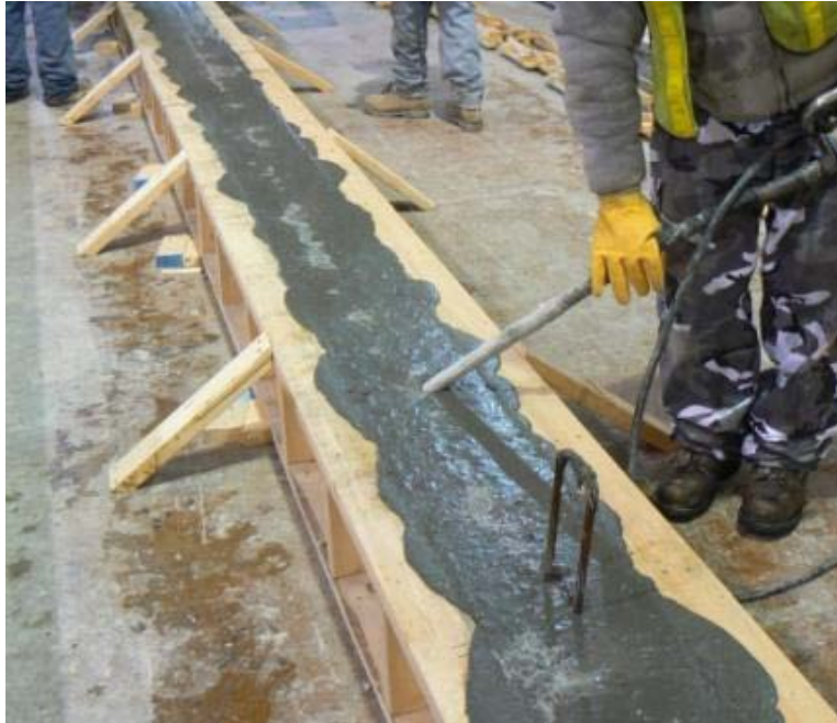
Figure 4.25. Vibrating freshly cast UHPC to ensure complete filling of forms
