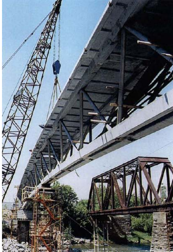
Figure 2.38. Placement of the second half segment of the Sherbrooke bridge on the falsework bent (Blais and Couture 1999)
