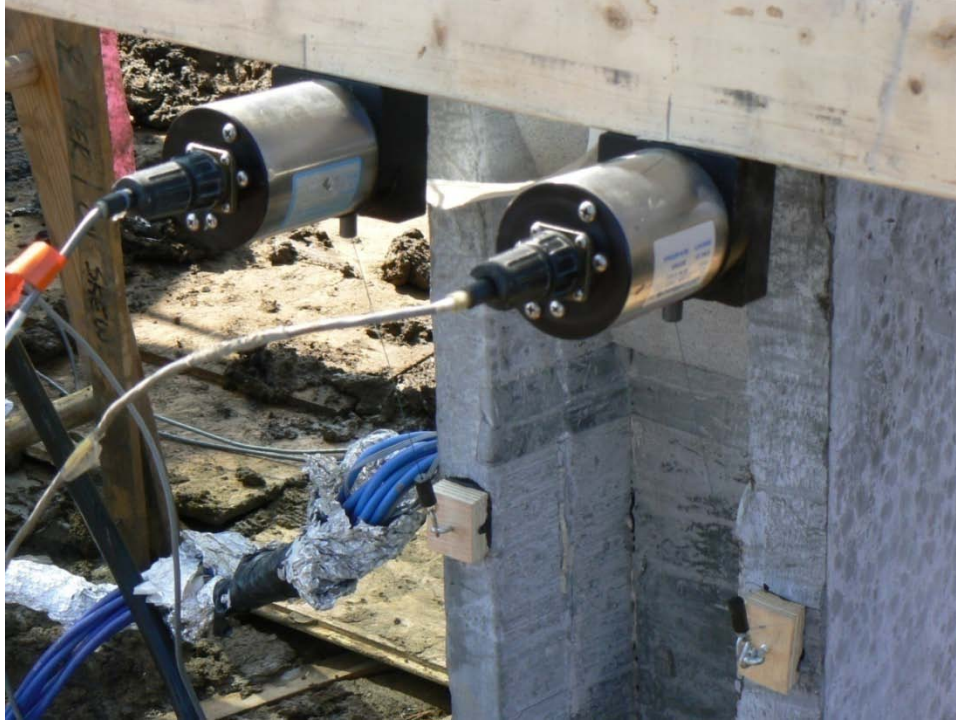
Figure 5.20. Displacement transducers and eye-hooks mounted to a UHPC pile
