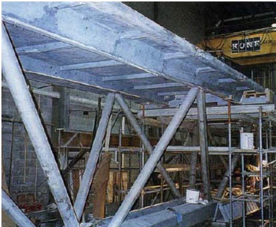
Figure 2.37. Sherbrooke bridge segment just after form removal (Blais and Couture 1999)
