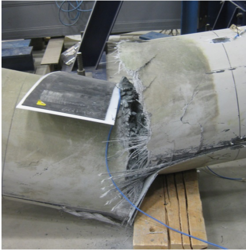
Figure 25: Tension Failure of Pile A-4FB
