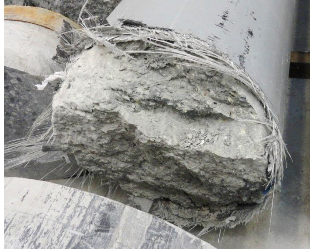
Figure 32: Cut at Failure of Pile E-4FB
