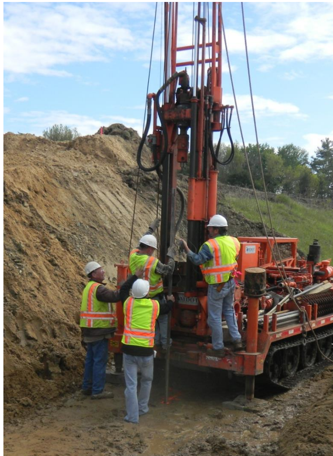
Figure 2-9 Installation of embedded sensors
