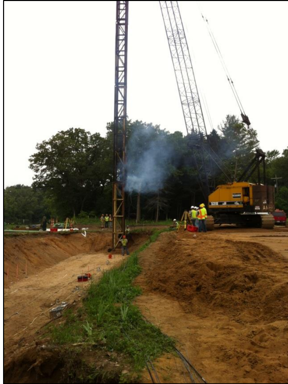
Figure 2-31 Driving test pile #37 at US-131 B site
