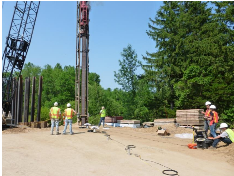
Figure 2-12 Pile driving at M-25 site
