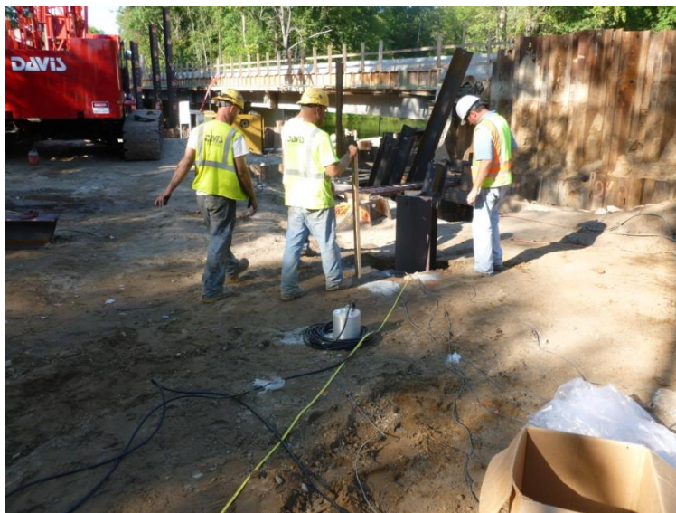
Figure 2-21 Test pile after end of pile driving at M-139 site
