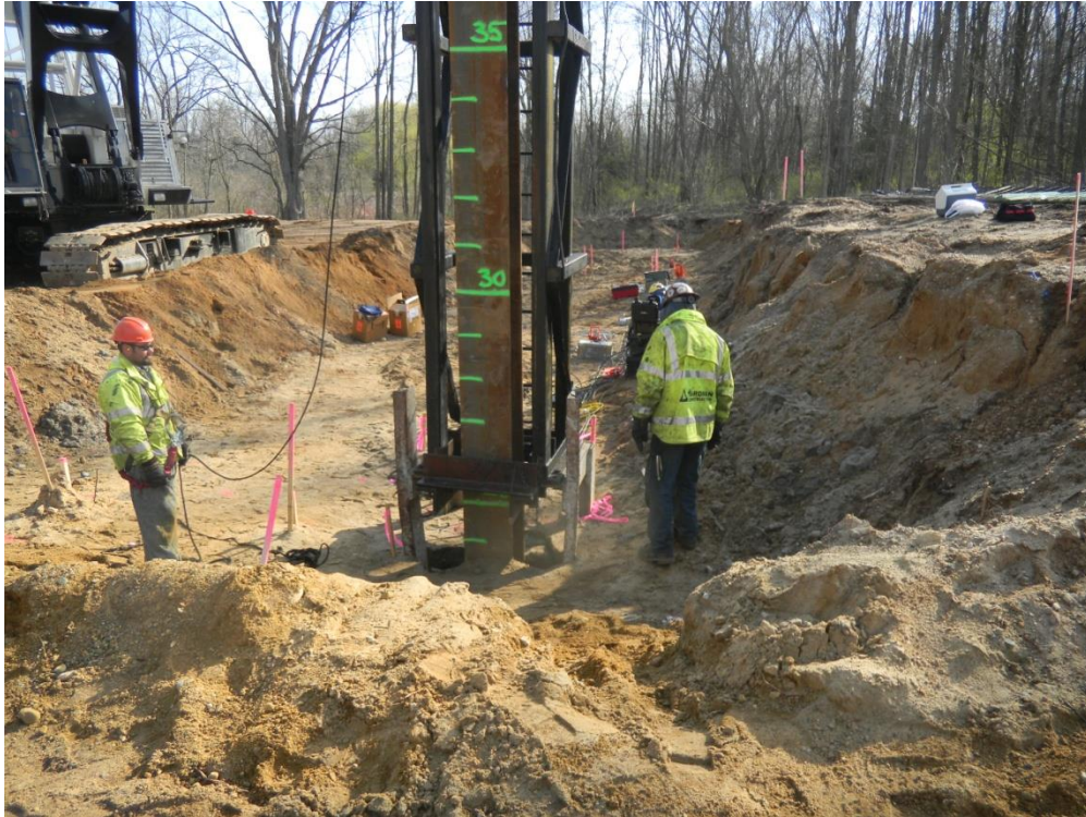
Figure 2-26 Driving test pile #1 at US-131 A site
