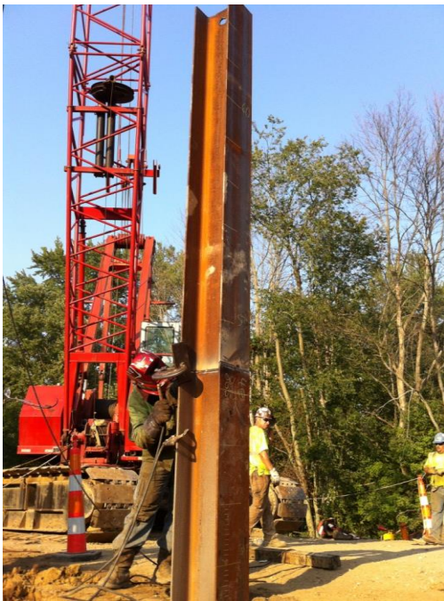
Figure 2-16 Welding second section of pile
