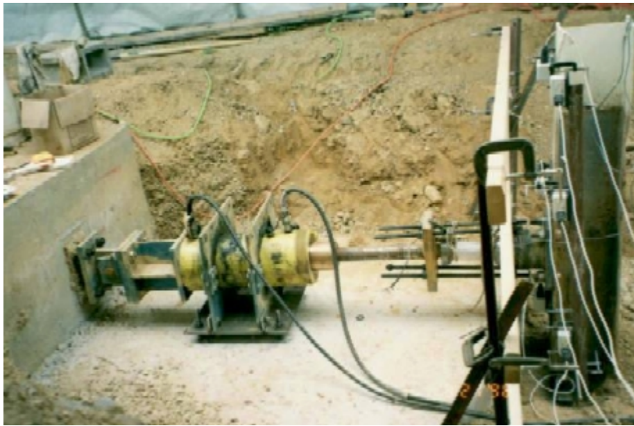
(b) Load test in progress at north pile.
