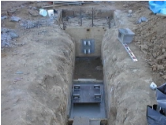
(c) Trench at setup A, ready for loading equipment.
