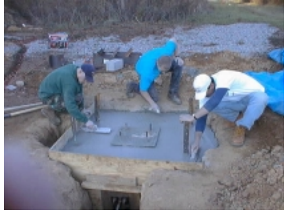
(b) Finishing concrete surface of 36" deep cap.
