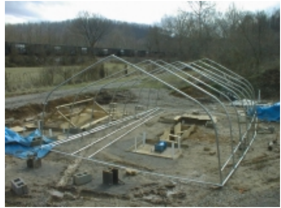
(b) Tent frame under construction.
