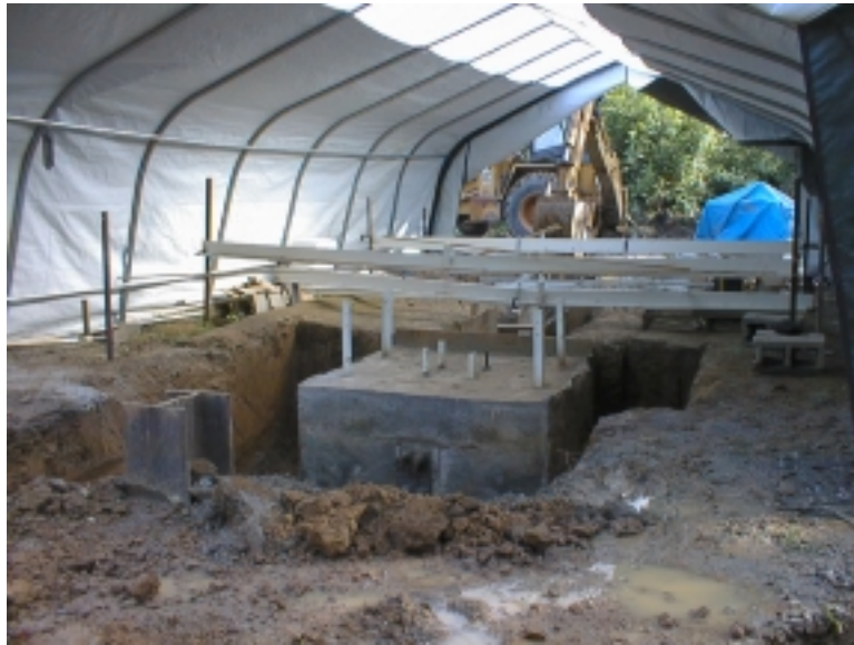
(a) Photograph of soil excavation around pile cap.
