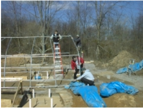
(a) Erecting tent frame.
