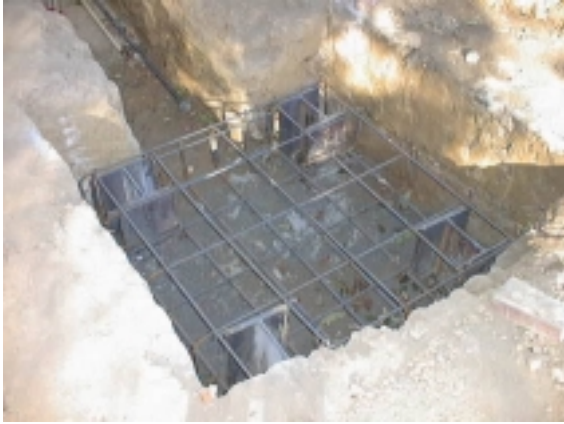
(a) Rebar in place for 18" deep cap.
