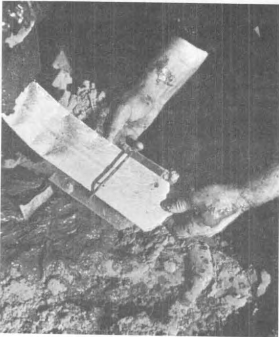
a. Placing the anchor on the drain
