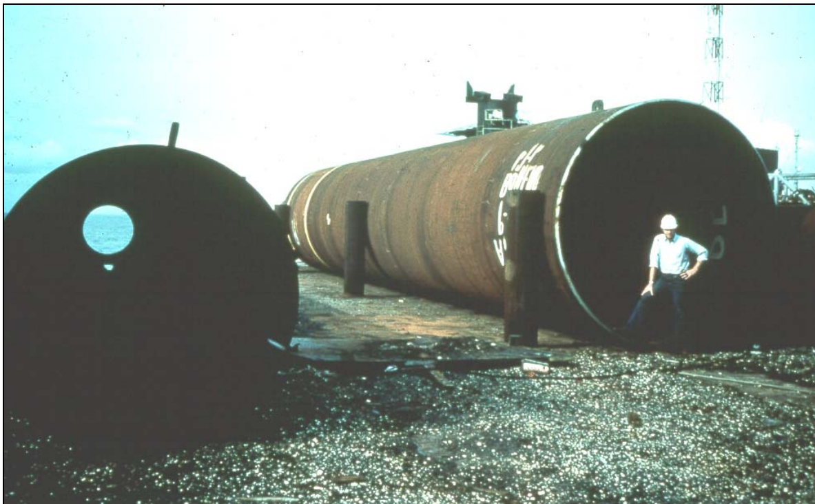
Figure 8.5 Large Diameter Open End Pipe Piles
