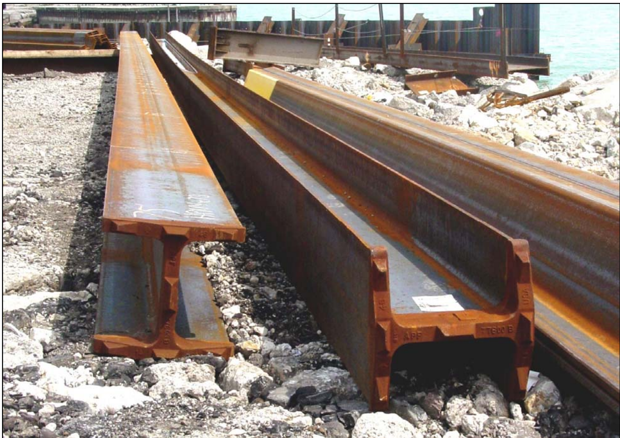
Figure 8.3 H-piles with Driving Shoes
