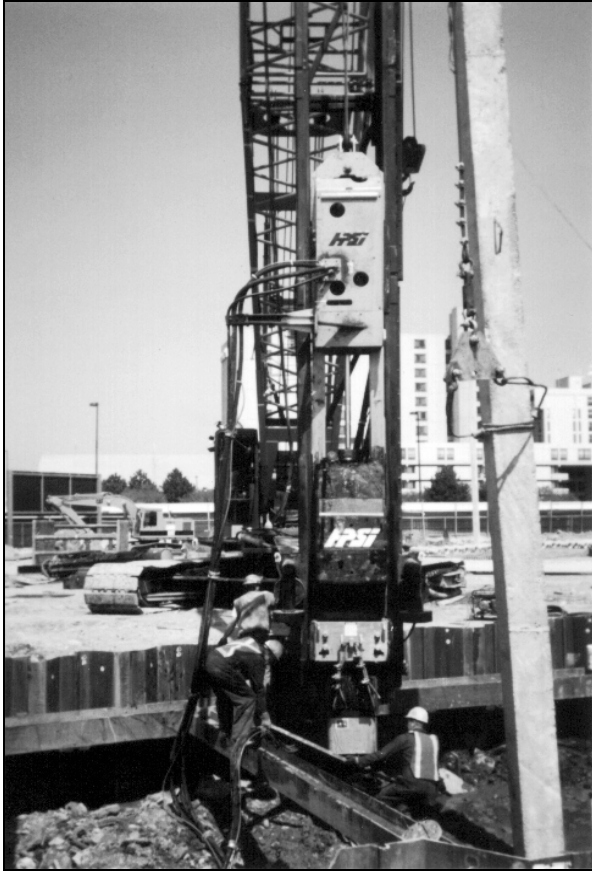
Figure 21.24 Single Acting Hydraulic Hammer
