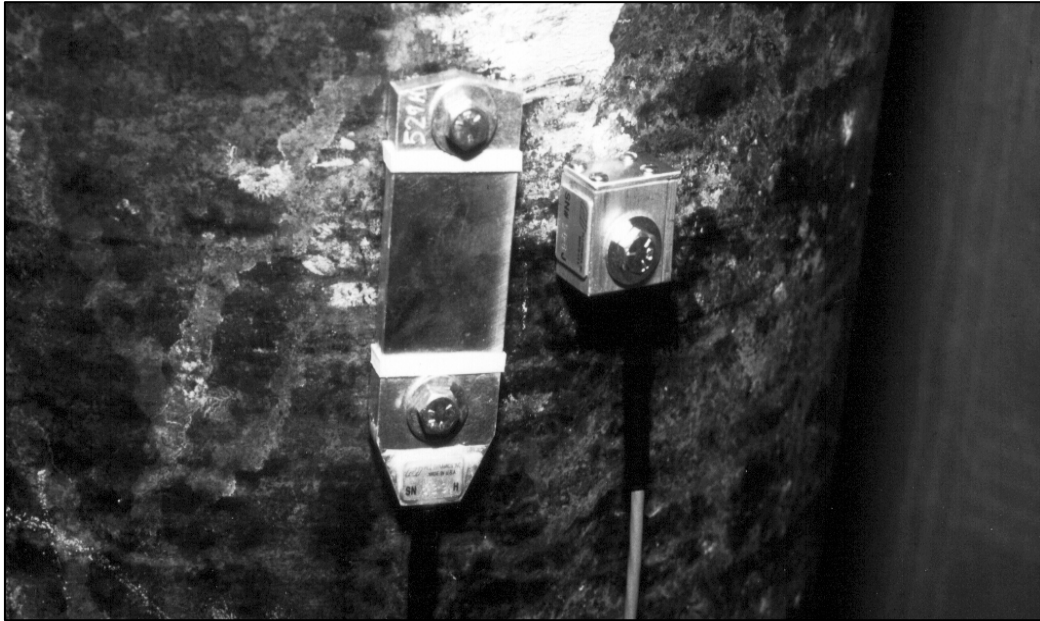
Figure 17.3 Strain Transducer and Accelerometer Bolted to Pipe Pile
