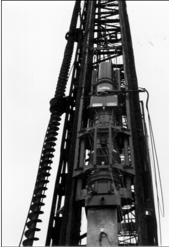
Figure 21.20 Single Acting Diesel Hammer (courtesy of Pileco)
