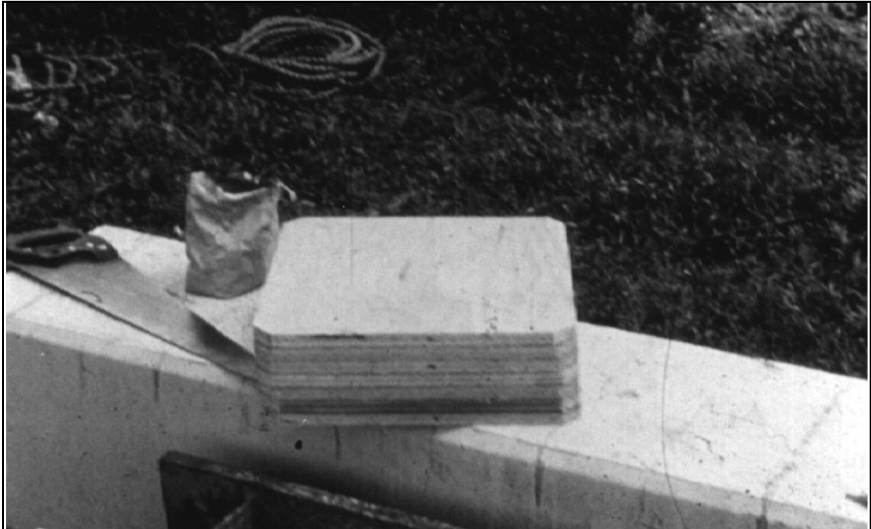
Figure 21.11 Plywood Pile Cushion
