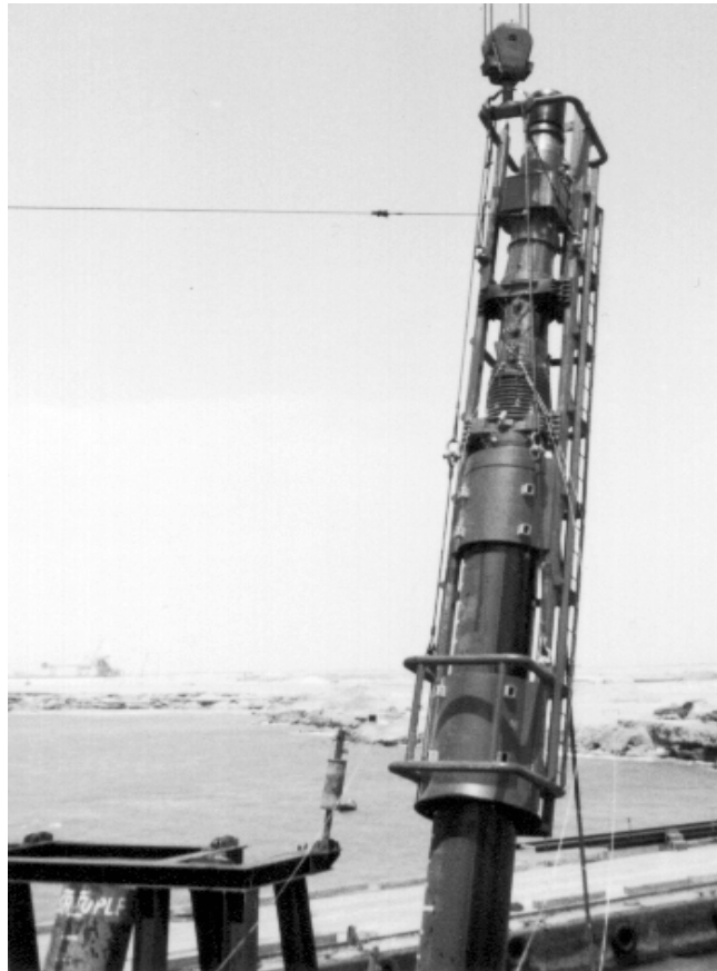
Figure 21.4 Typical Offshore Lead Configuration
