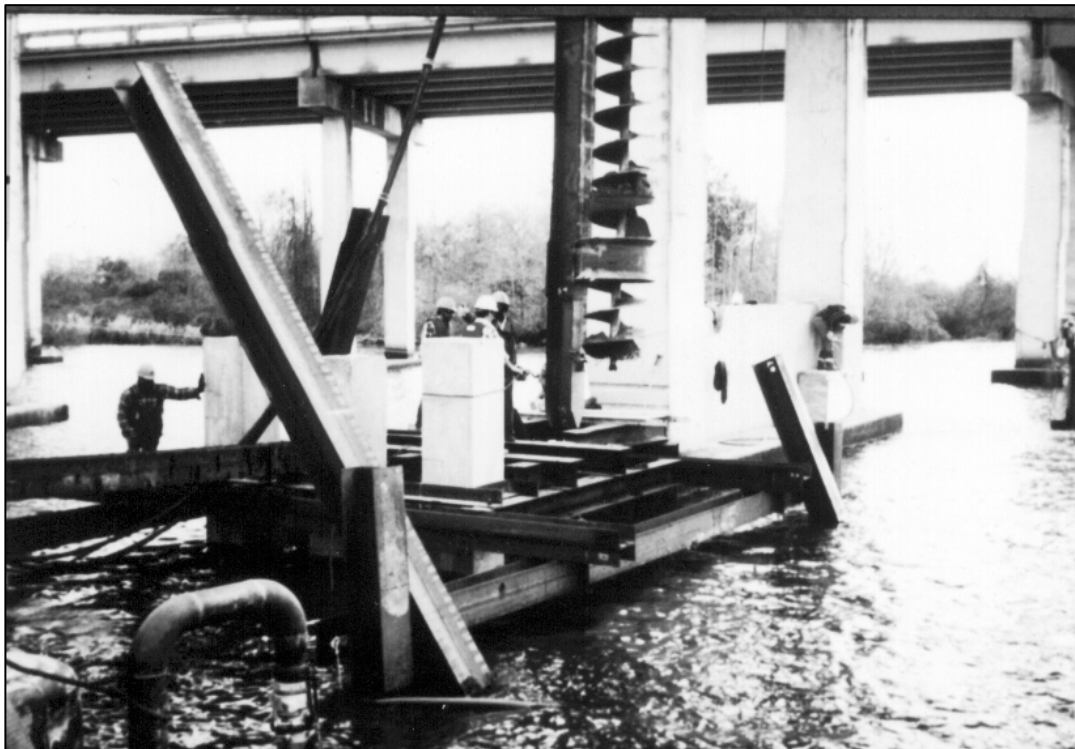
Figure 21.36 Solid Flight Auger Predrilling System (courtesy of Florida DOT)
