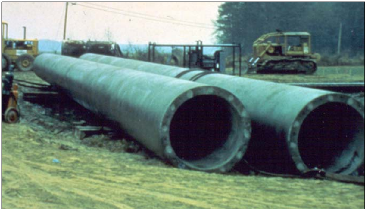
Figure 8.11 Concrete Cylinder Pile
