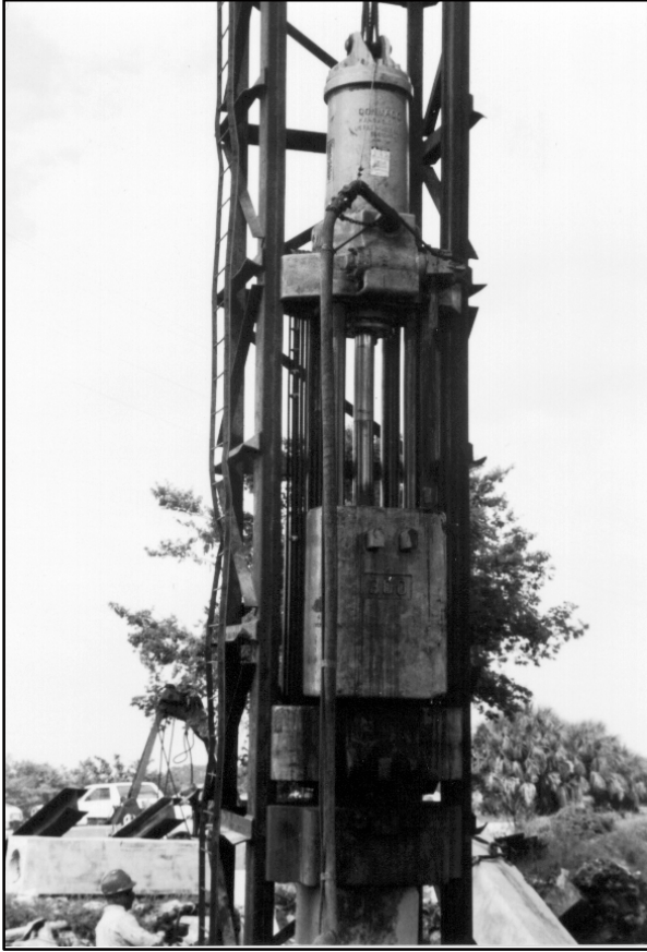
Figure 21.15 Single Acting Air Hammer
