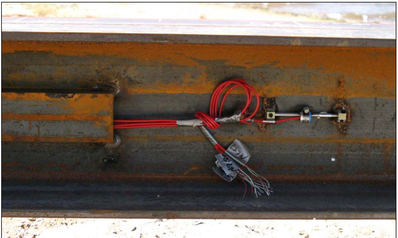
Figure 18.10 Arc-weldable Vibrating Wire Strain Gage Attached to H-pile. (Note: Protective Channel Cover Shown on Left)
