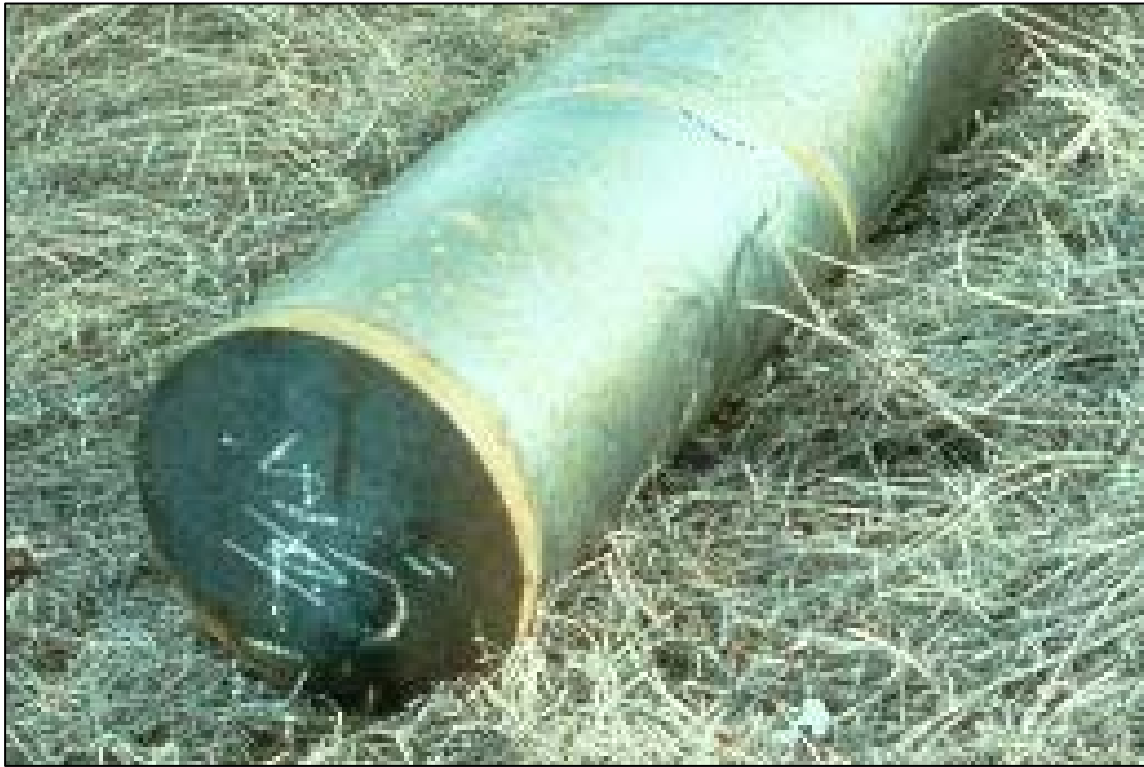
Figure 8.4 Typical Closed-End Pipe Pile
