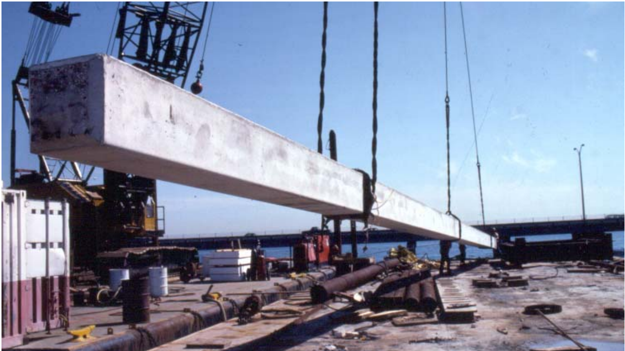
Figure 8.8 Square Prestressed Concrete Pile
