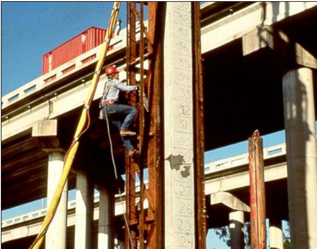
Figure 17.2 Pile Positioned for Driving and Gage Attachment
