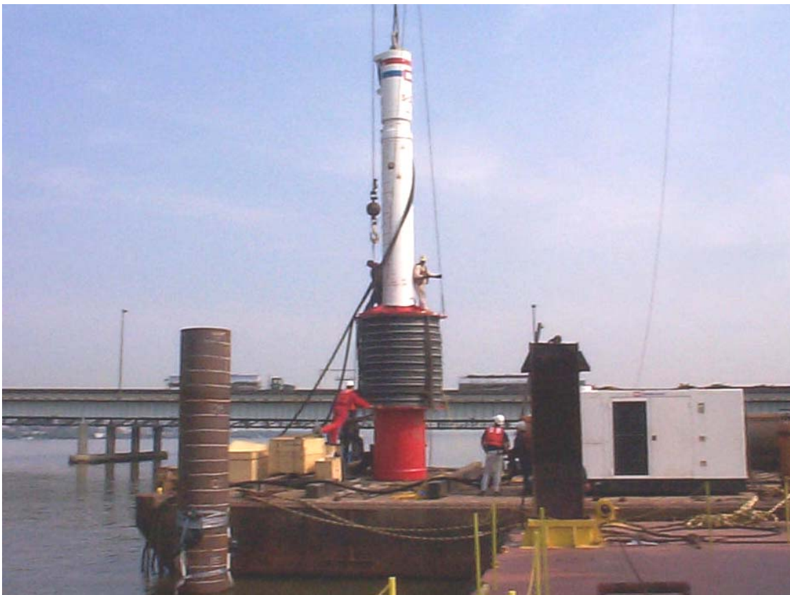
Figure 21.32 Noise Shroud for IHC Hydraulic Hammer
