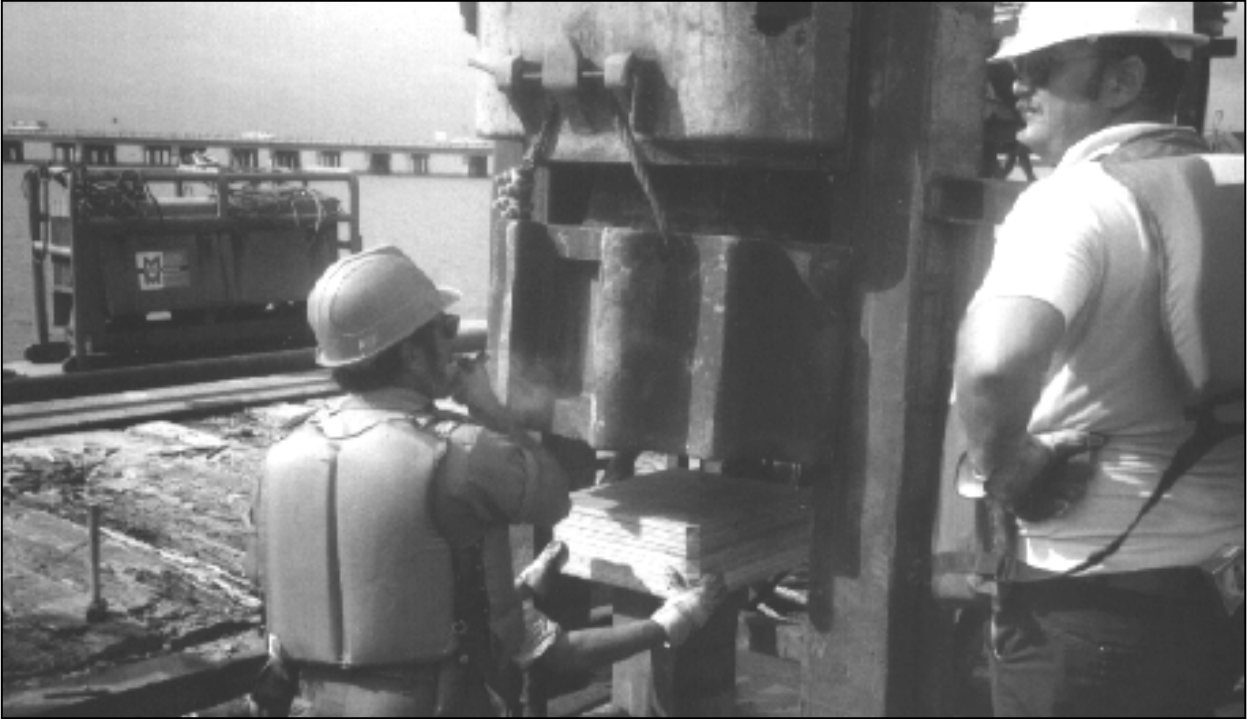
Figure 23.4 Pile Cushion Replacement
