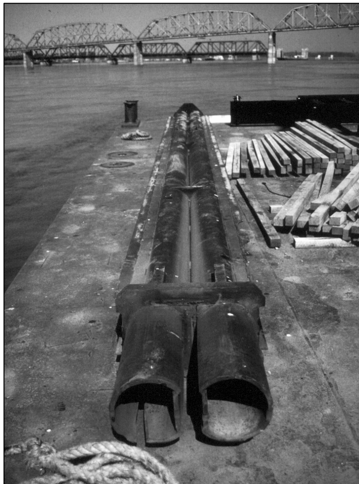
Figure 21.33 Follower used for Driving H-piles
