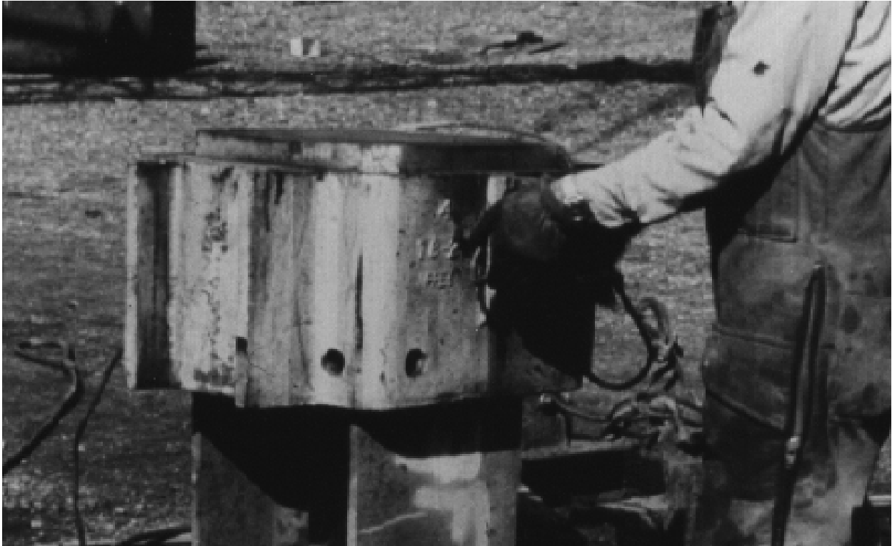
Figure 21.9 Helmet on H-pile
