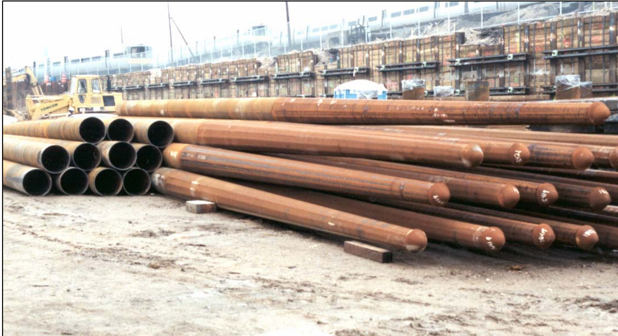
Figure 8.14 Tapered Tube Pile
