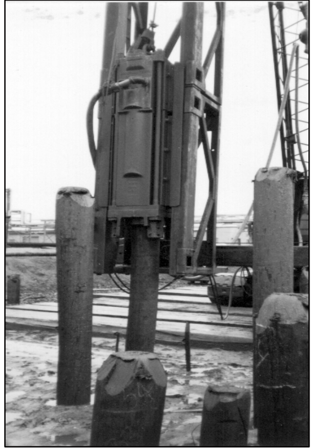
Figure 21.16 Double Acting Air Hammer
