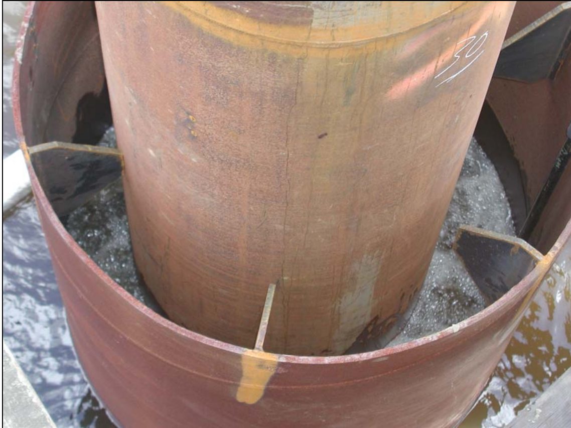
Figure 21.37 Bubble Ring with Containment Device (courtesy WSDOT)
