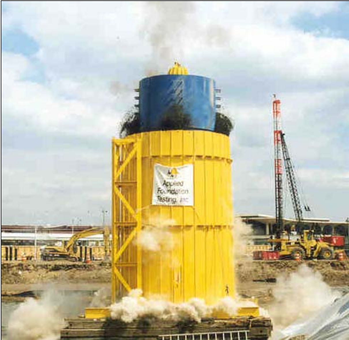
Figure 20.3. STATNOMIC test in progress with gravel catch mechanism 40,000 kN (9,000 kip) device. (courtesy of Applied Foundation Testing)
