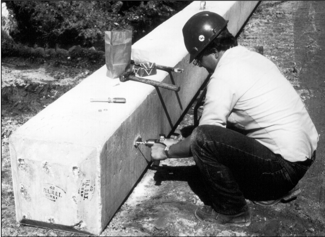
Figure 17.1 Pile Preparation for Dynamic Testing
