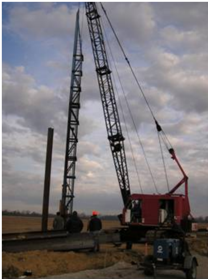
Figure A.4 ICE-42S diesel hammer used in pile driving
