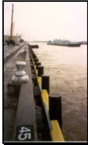
Figure 5. Photo. Fendering system, Nashville Avenue Marine Terminal, Port of New Orleans, LA.
