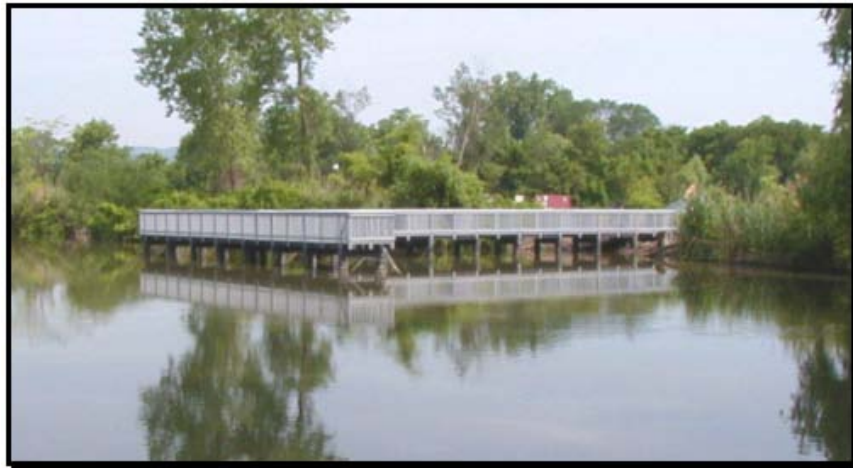
Figure 6. Photo. Floating dock project.
