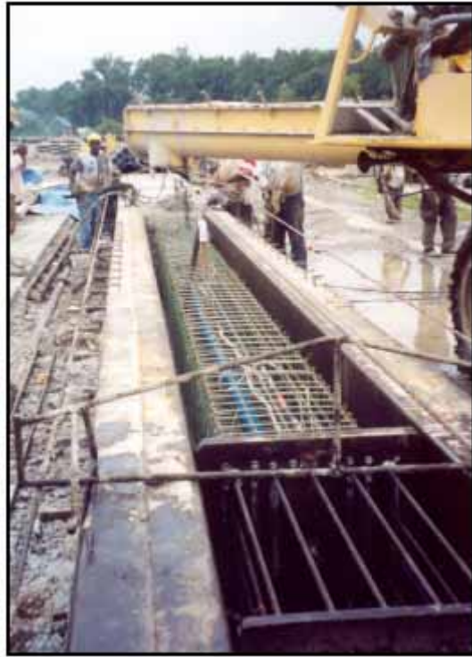
Figure 85. Photo. Fabrication of prestressed concrete pile.
