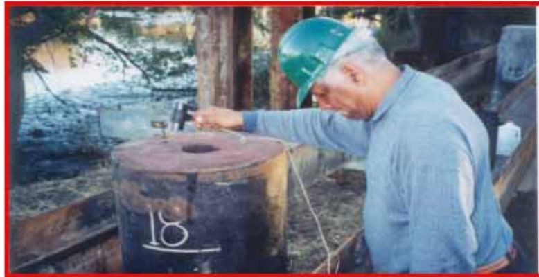
a) PIT on plastic pile after installation
