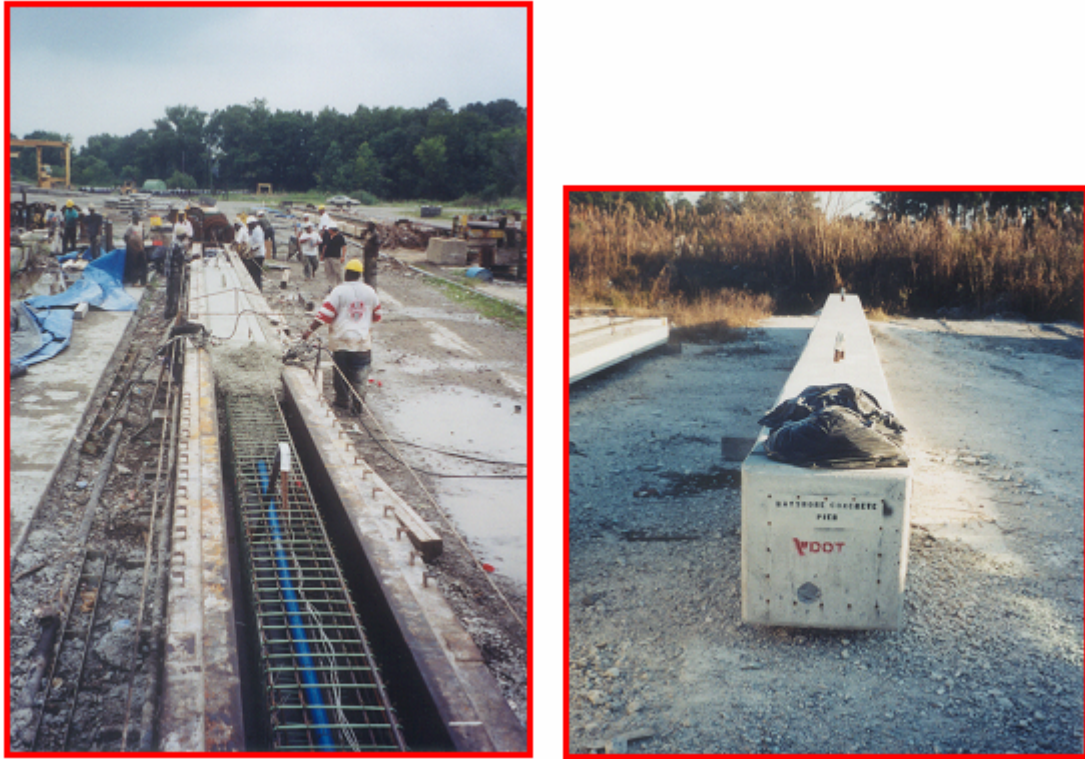
Figure 120. Photos. Fabrication of prestressed concrete test pile.
