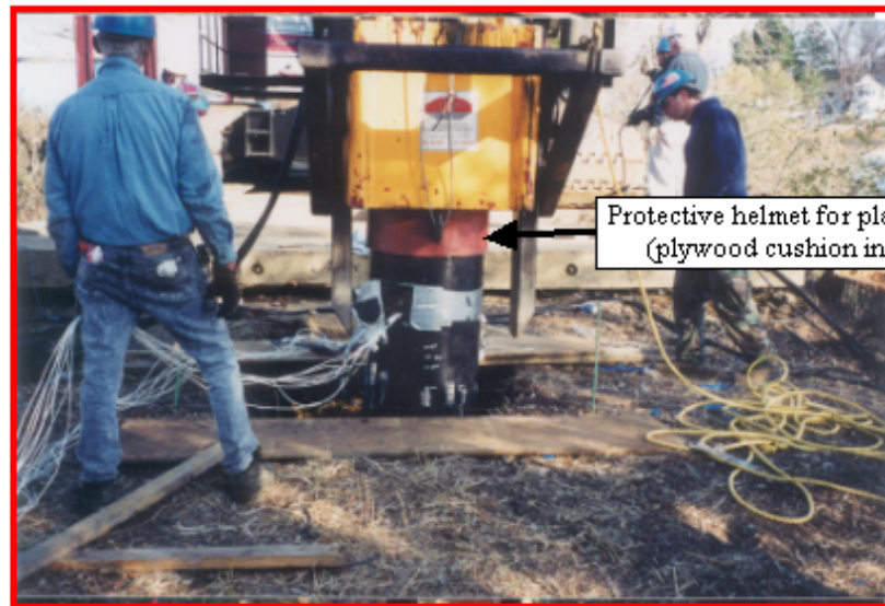
c) Restrike of plastic pile
