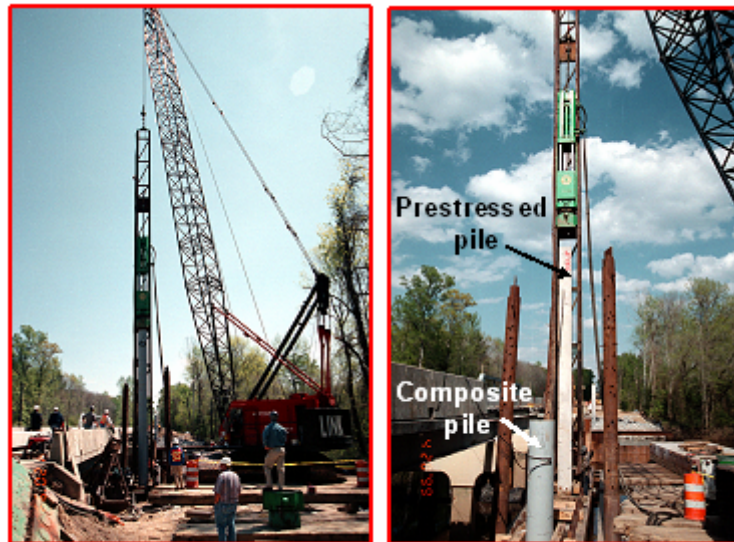
a) Driving of composite pile
