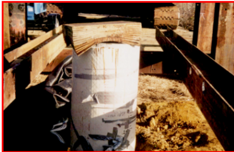
c) End of driving of FRP pile showing driving cushion compressed
