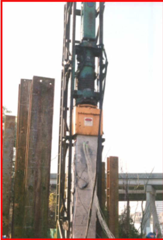
a) Driving of prestressed pile
