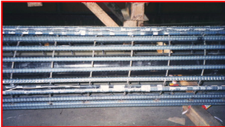
Figure 124. Photos. Rebar cage of the plastic composite test pile.
