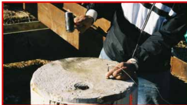
c) PIT on FRP pile after installation
