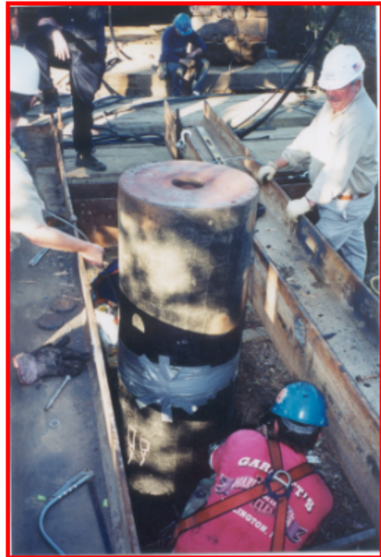
b) End of driving of plastic pile
