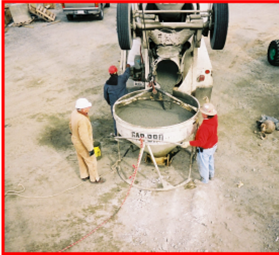
(a) Concrete is poured into bucket
