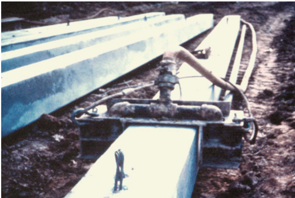
Figure 15-46 Dual jet system mounted on concrete pile (courtesy of Florida DOT).
