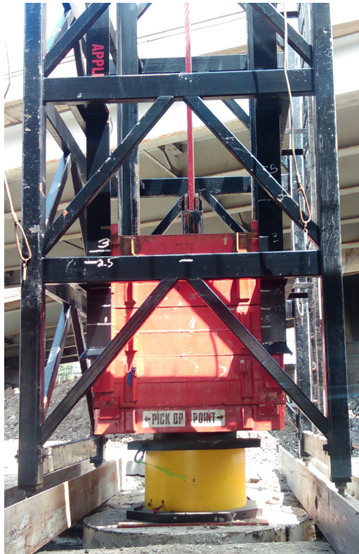
Figure 11-8 APPLE 32 ton modular rapid load test system with transducer.
