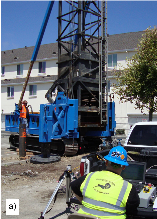
Figure 11-7 Drop weight rapid load test systems: (a) Fundex system (courtesy Foundation Constructors Inc.) and (b) Hybridynamic system.
