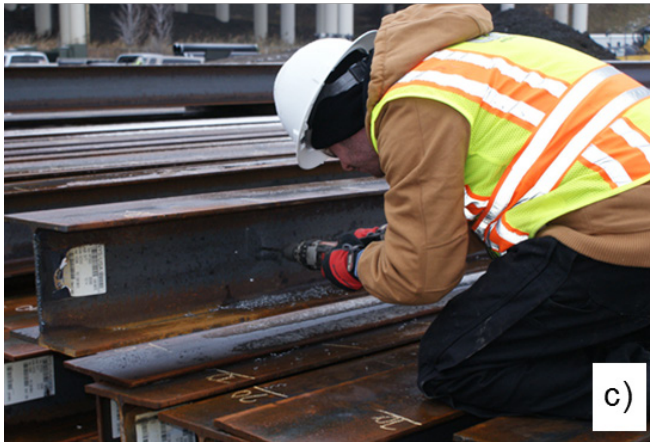
Figure 10-1 Pile preparation for dynamic testing.
