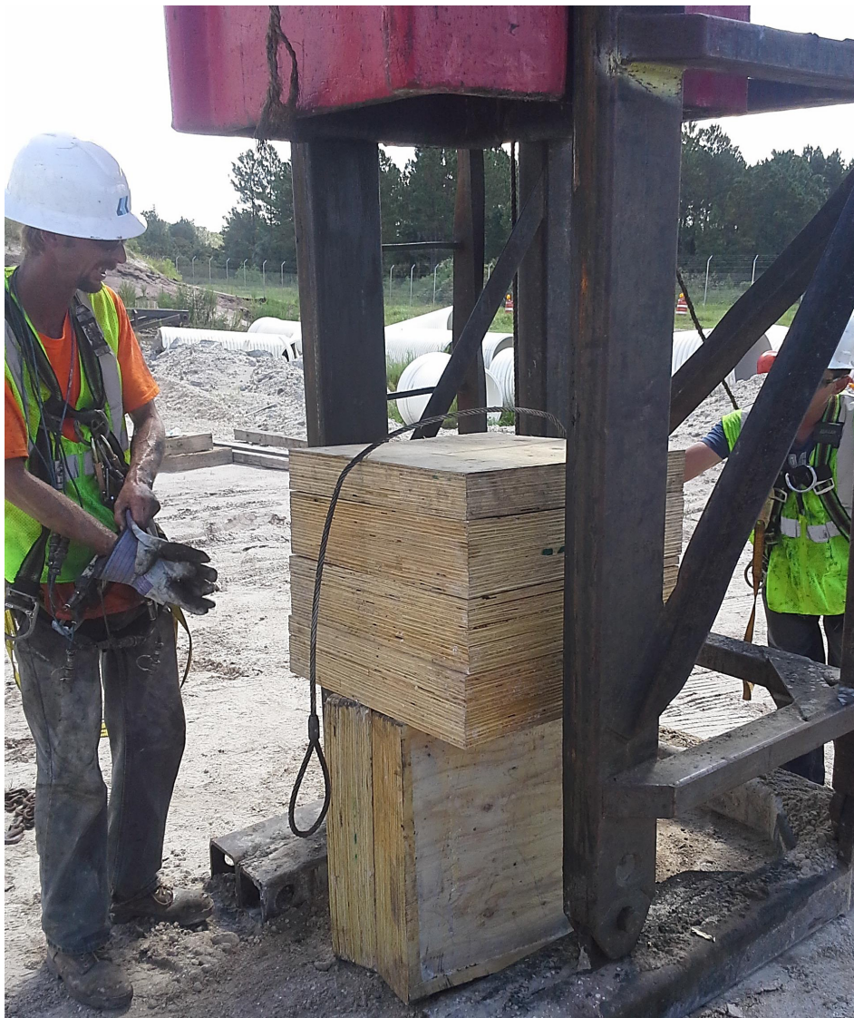
Figure 18-5 New pile cushion being inserted into helmet.
