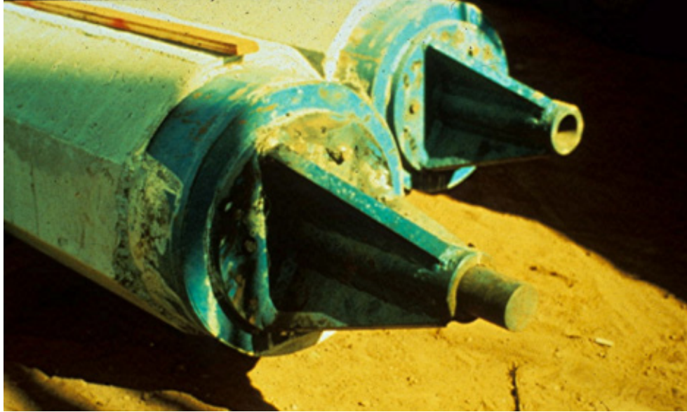
Figure 16-25 Oslo point for concrete pile.
