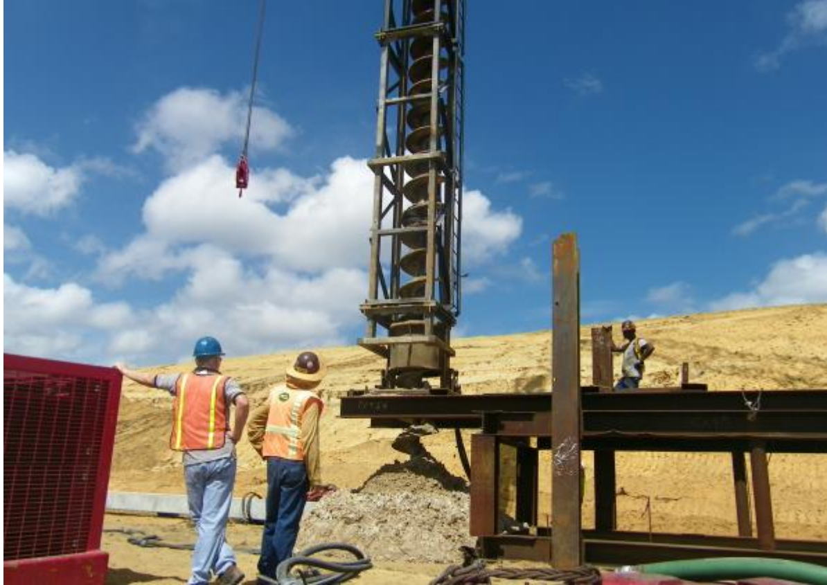
Figure 15-48 Solid flight auger predrilling system.
