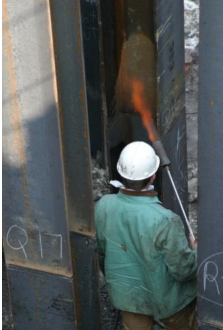
Figure 16-41 Heating pile splice location prior to welding.
