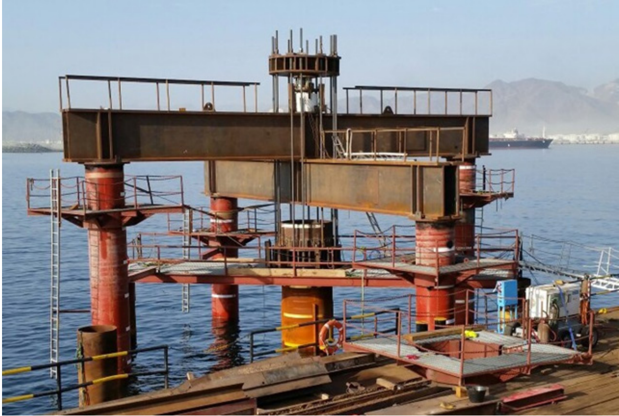
Figure 9-9 Tension test on pipe pile using reaction piles (courtesy of Besix).
