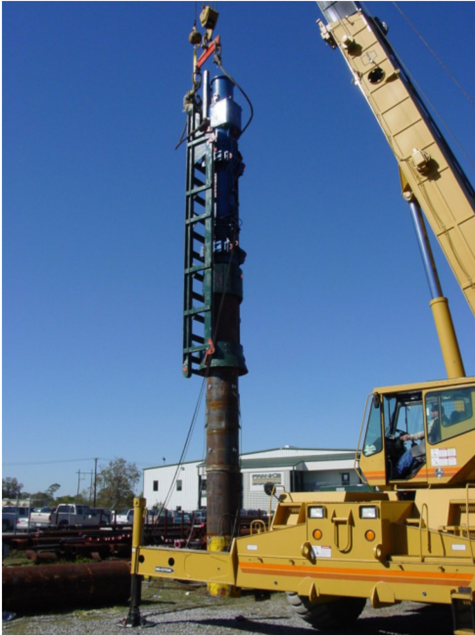
Figure 15-3 Rough terrain pile driving rig with telescoping boom and offshore leads.
