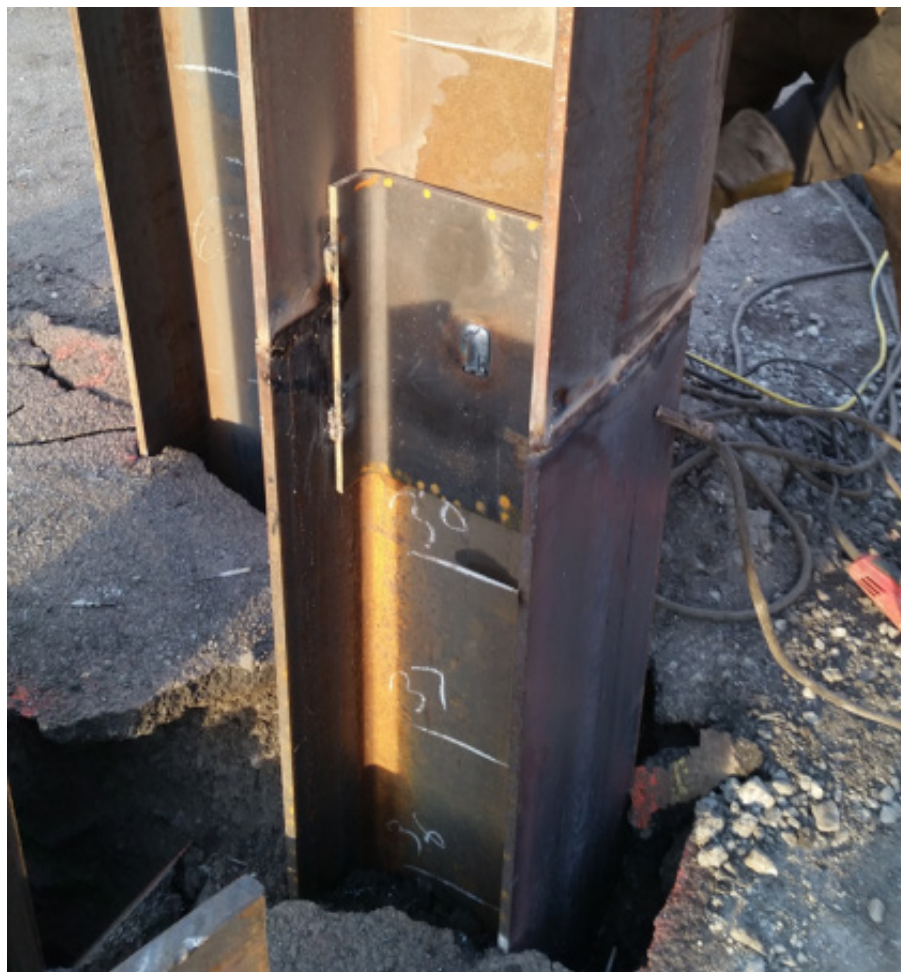
Figure 16-9 Partially completed splice using H-pile splicer.
