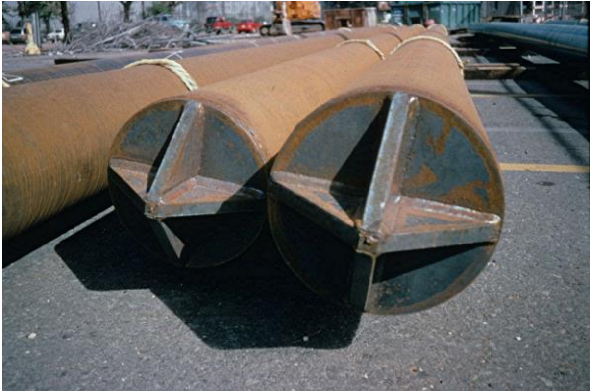
Figure 16-13 Rock crusher driving shoe welded on a closed end steel pipe pile.
