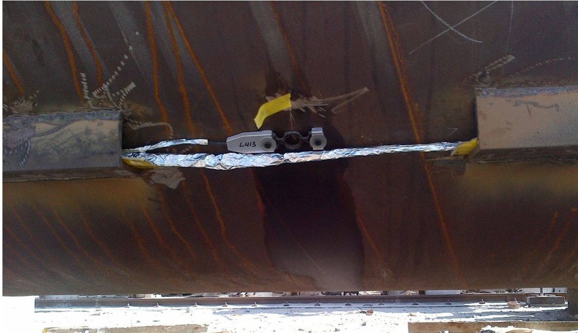
Figure 9-23 Waterproof electrical resistance strain gage bolted on pipe pile with protective channel (courtesy of Besix).
