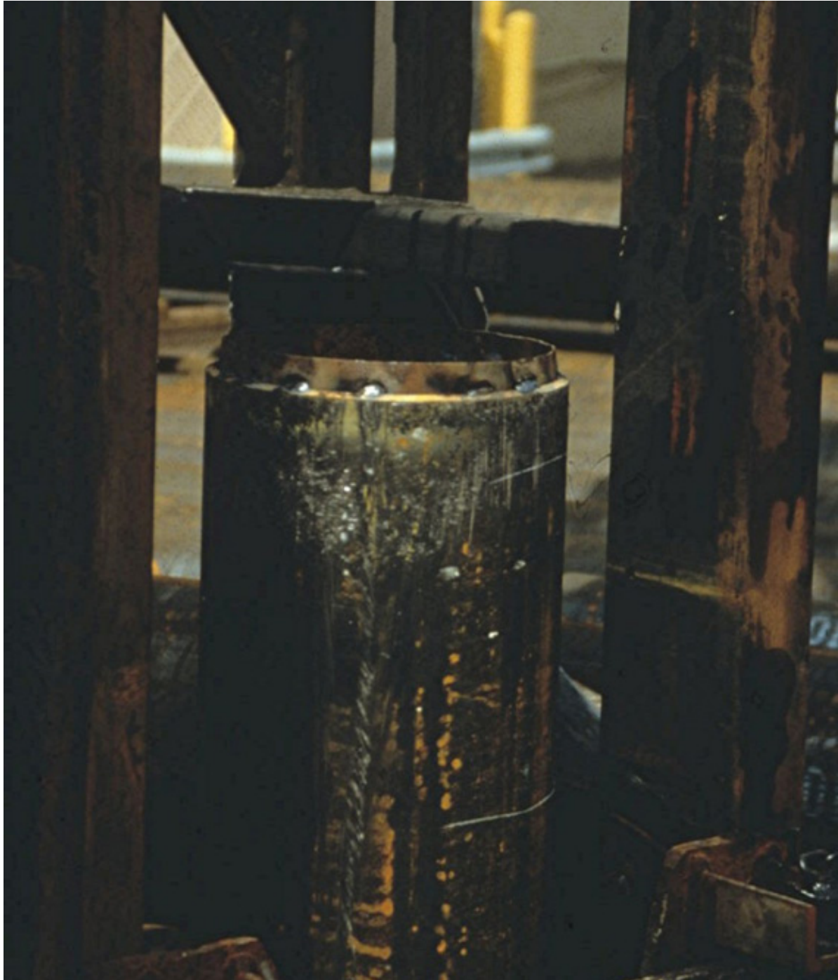
Figure 16-19 Backing ring tack welded to bottom pile.
