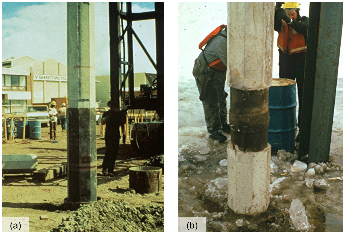
Figure 16-33 Sleeve splices: (a) Hawaiian can and (b) Bruns splice.
