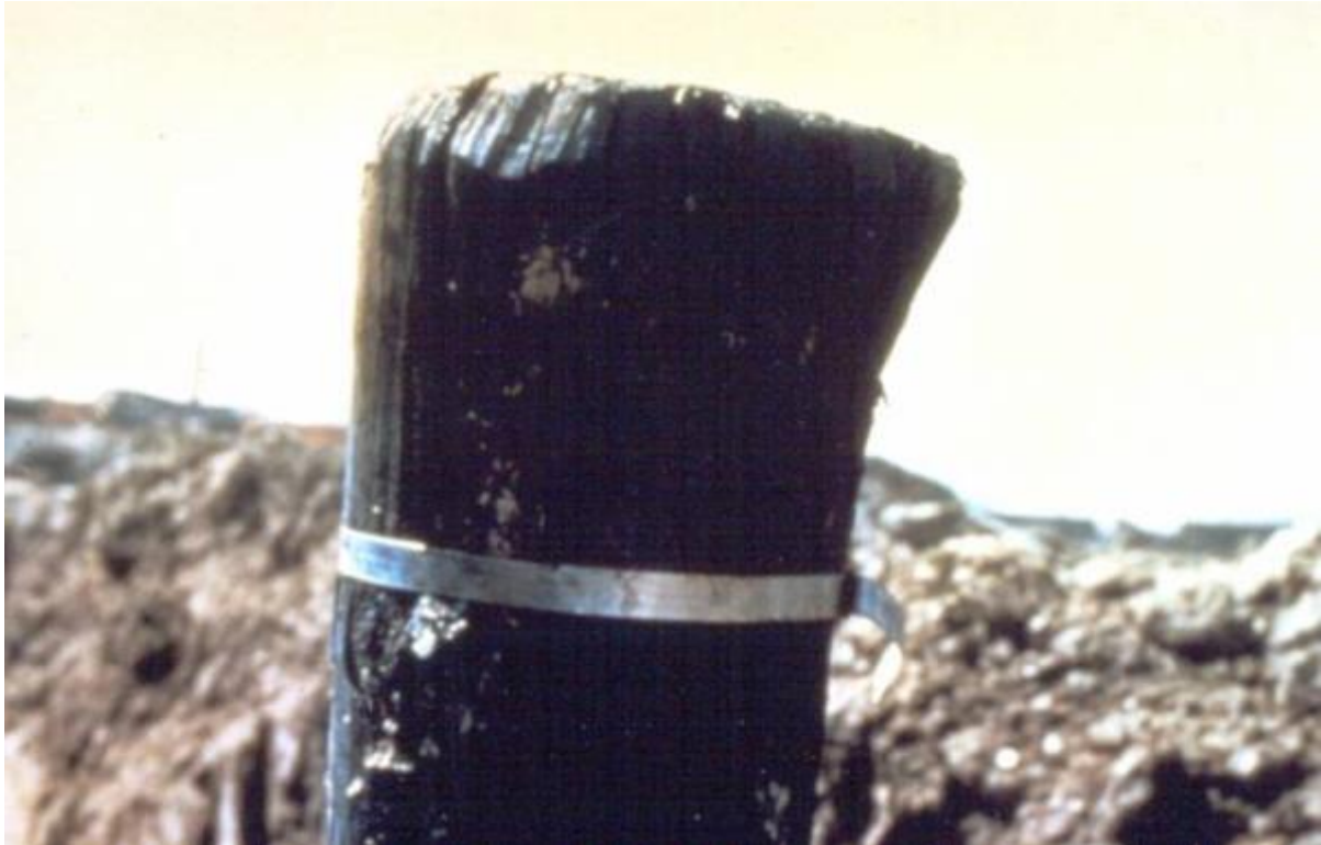
Figure 16-3 Banded timber pile head.
