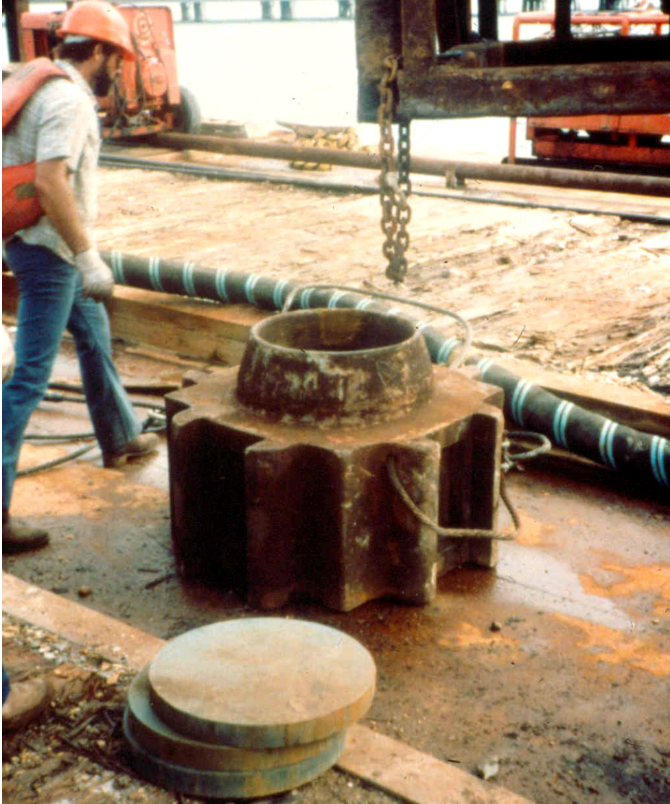
Figure 18-3 Check of Blue Nylon hammer cushion material before use.
