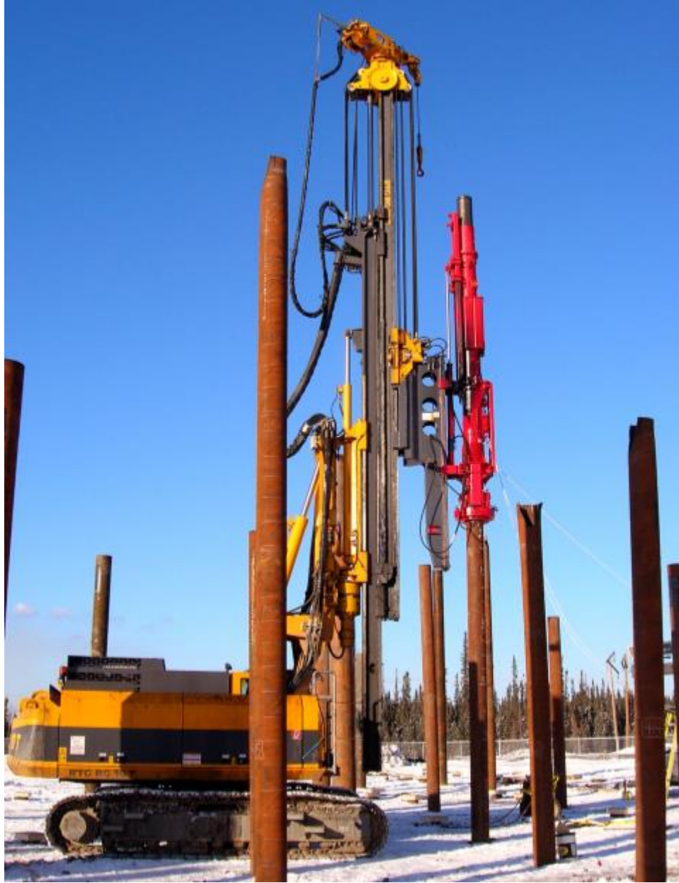
Figure 15-5 Universal rig setup for pile driving (courtesy Bauer-Pileco).
