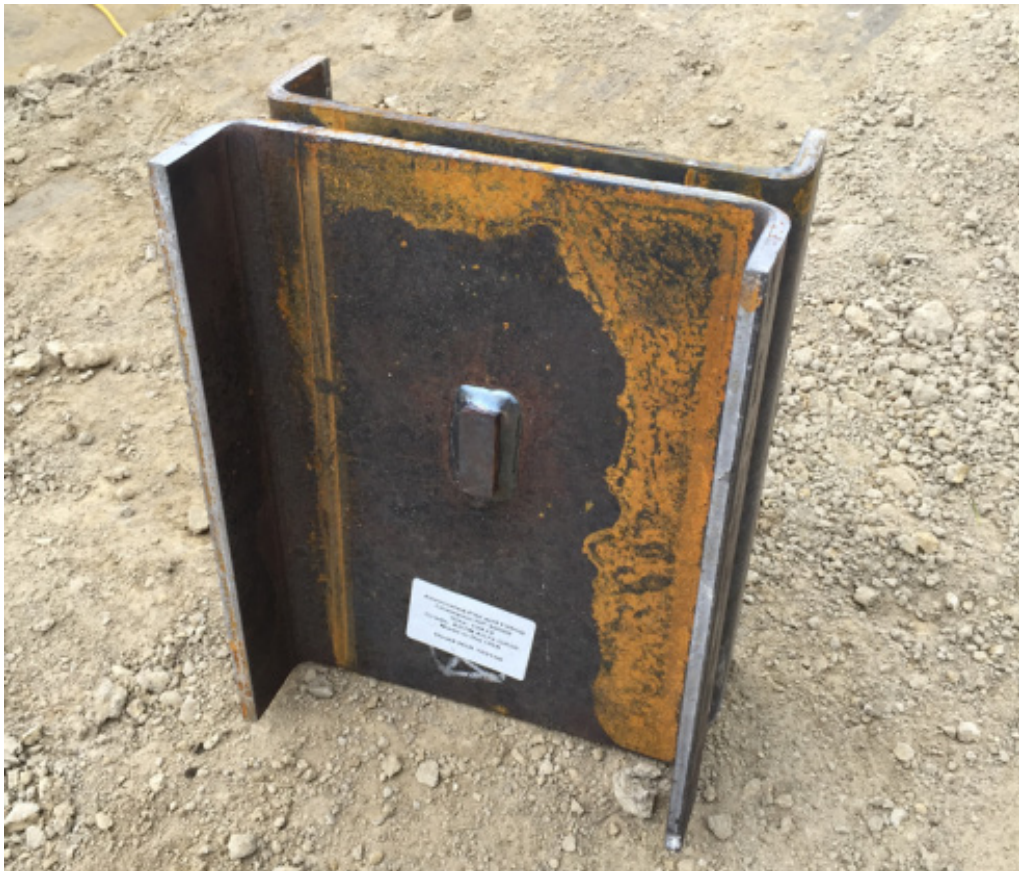
Figure 16-8 H-pile splicer.
