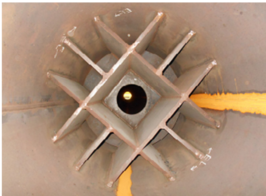
Figure 6-15 Constrictor plate installed inside pipe pile.
