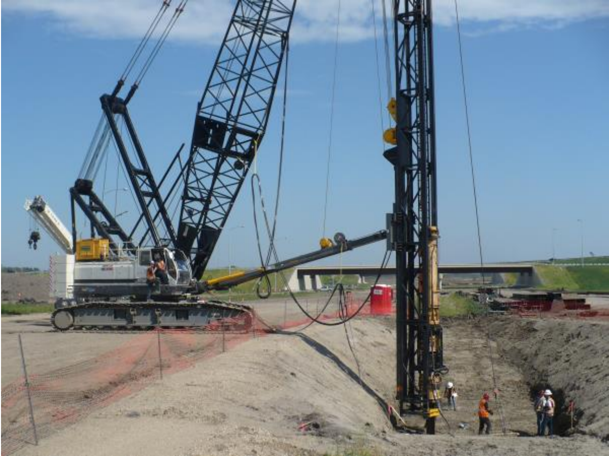
Figure 15-12 Vertical travel lead system (courtesy Berminghammer).
