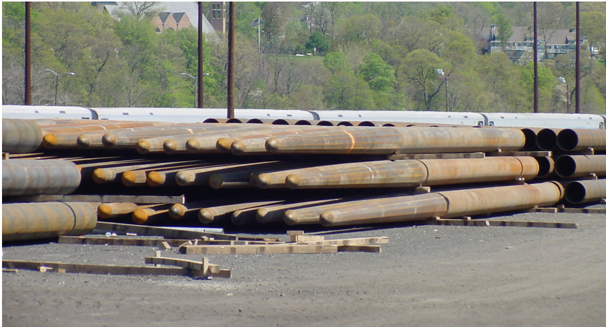
Figure 6-17 Tapertube piles (courtesy DFP Foundation Products, LLC).
