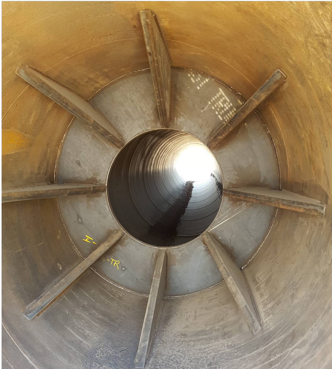
Figure 16-23 Constrictor plate installed inside pipe pile.
