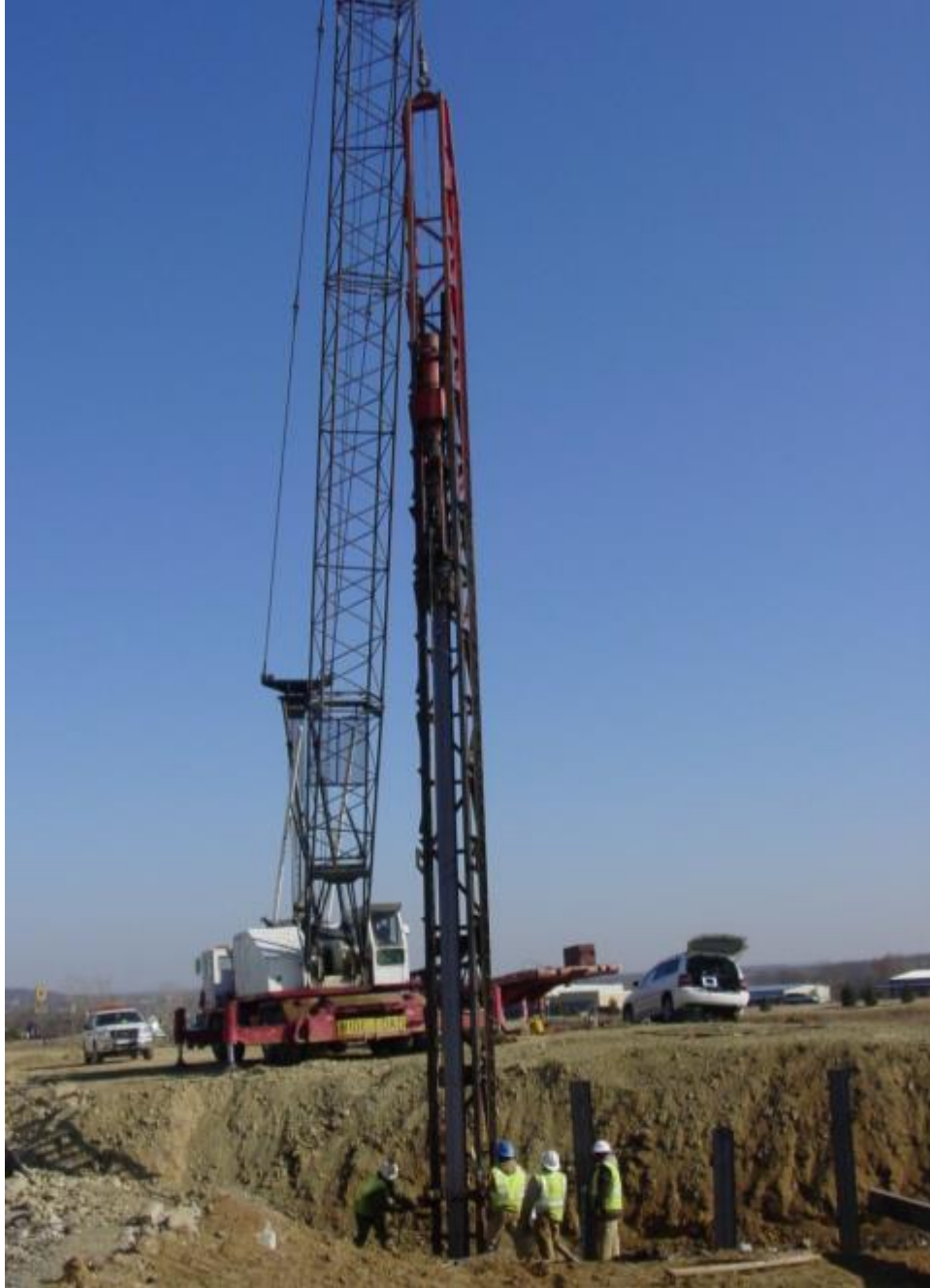
Figure 15-2 Truck crane pile driving rig with lattice boom and swinging leads.
