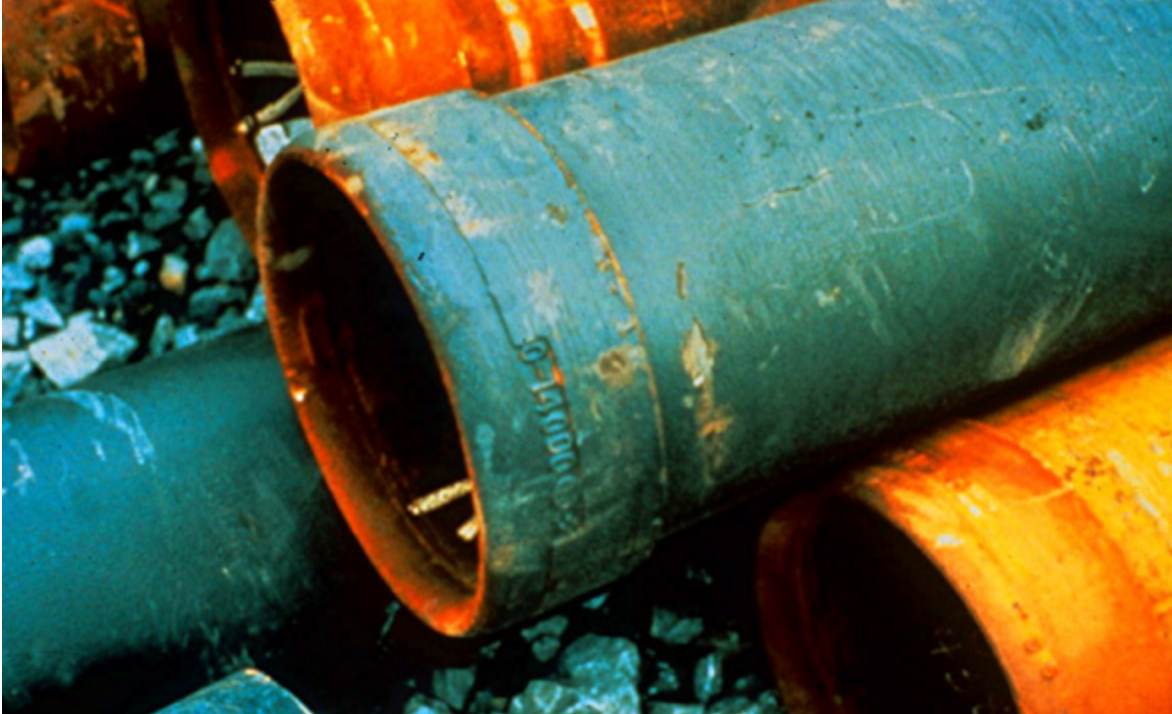
Figure 16-16 Outside flange cutting shoe on open end steel pipe pile.
