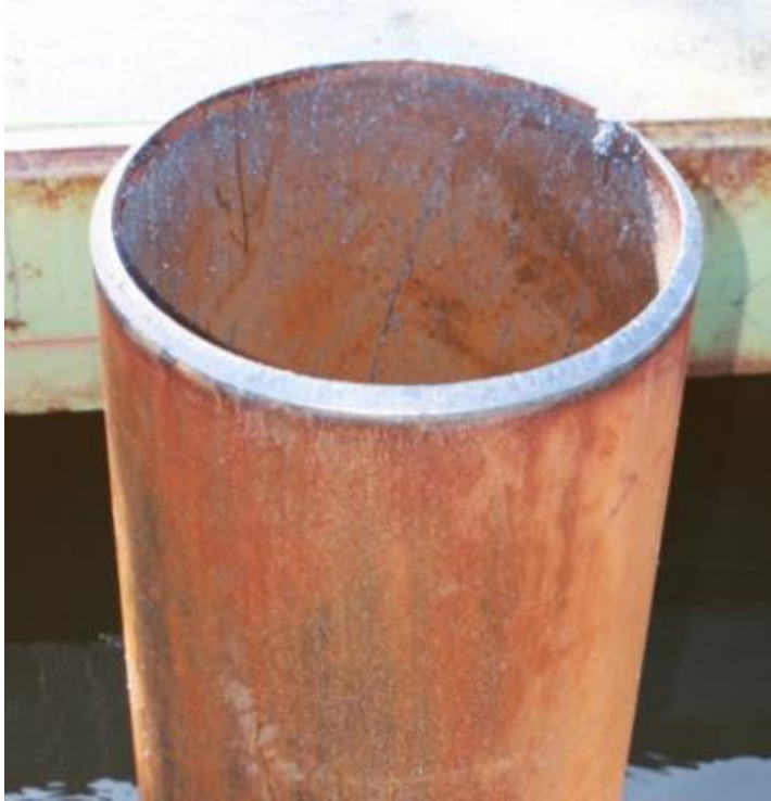
Figure 16-36 Beveled edges on pipe pile in preparation for weld.
