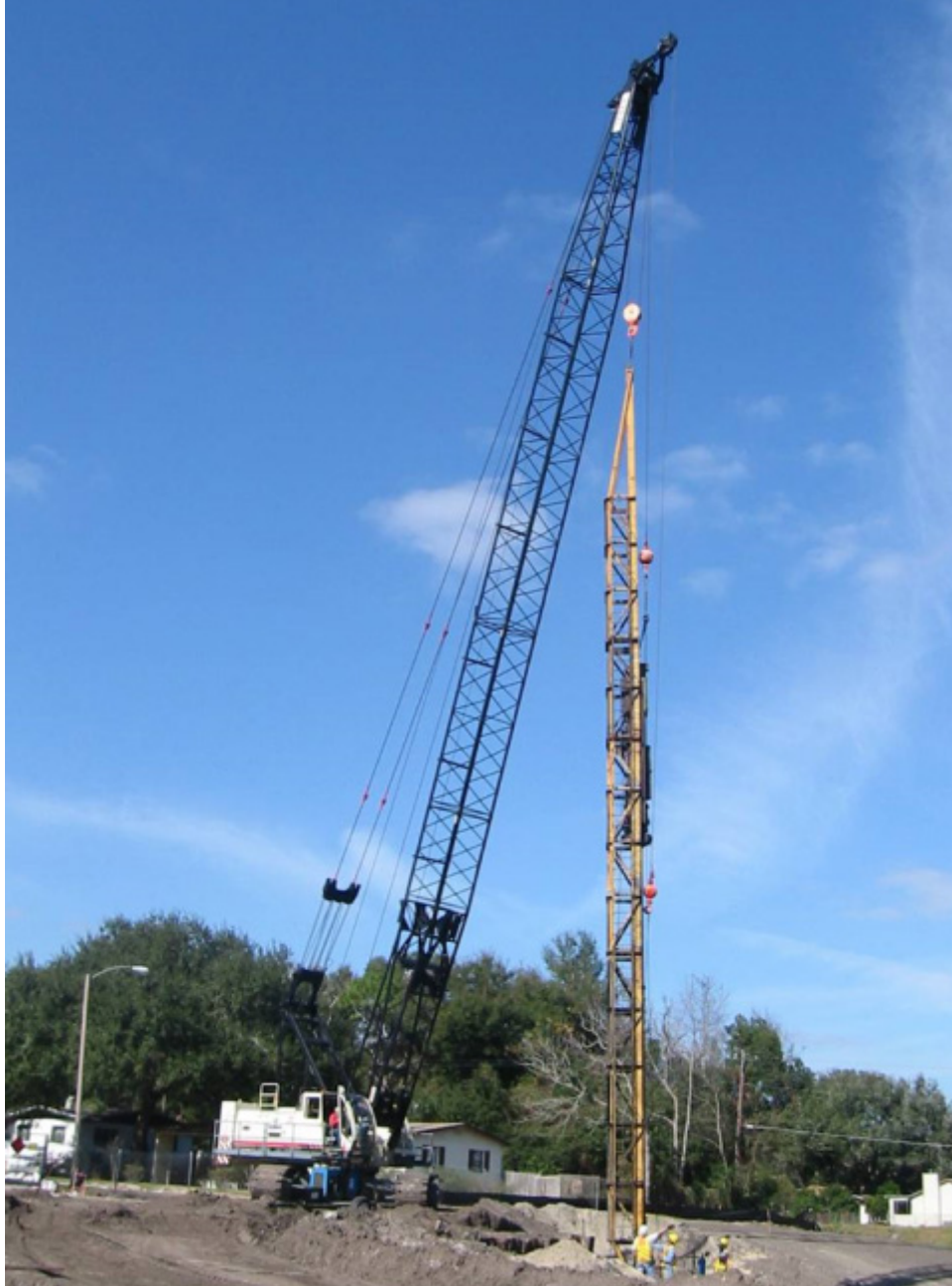
Figure 15-1 Crawler crane pile driving rig with lattice boom and swinging leads.
