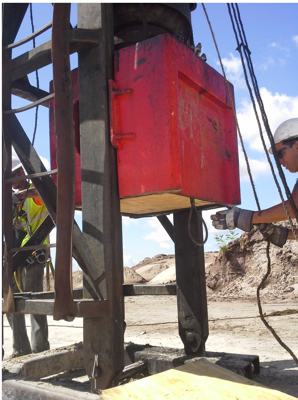
Figure 18-6 Helmet with new pile cushion installed.
