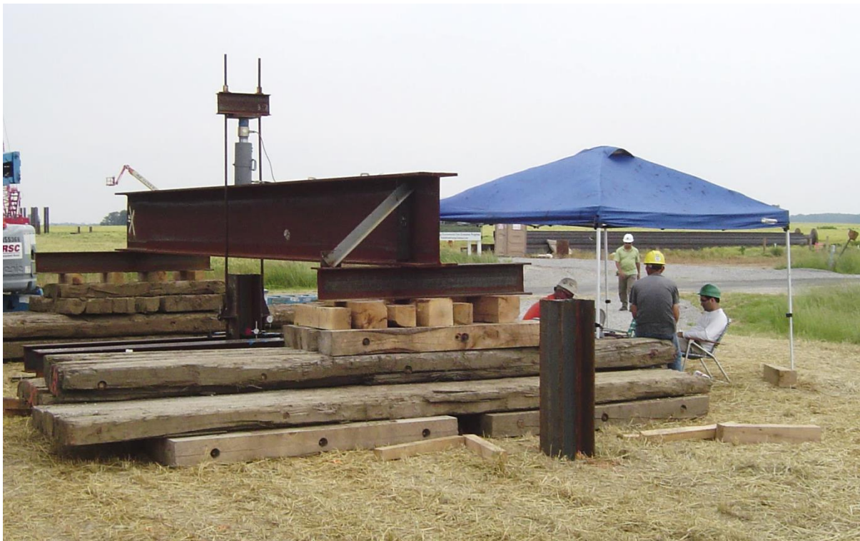
Figure 9-10 Tension test on H-pile using mats and cribbing (courtesy of WKG 2 ).
