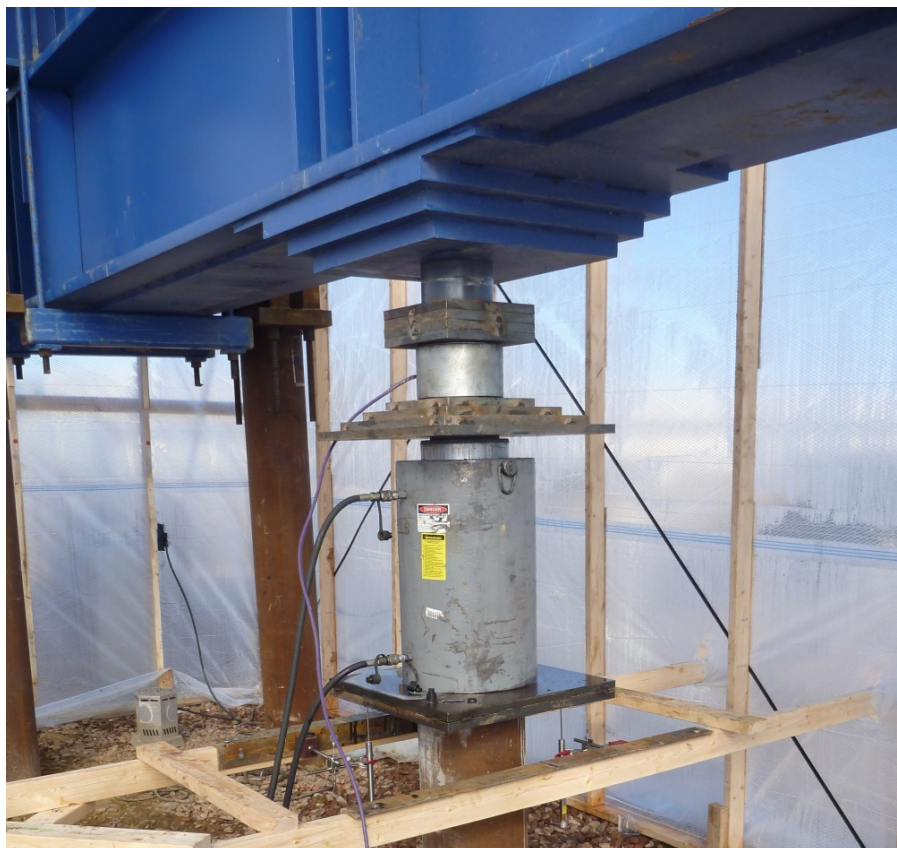
Figure 9-5 MnDOT reaction beam and load test setup (courtesy MnDOT).
