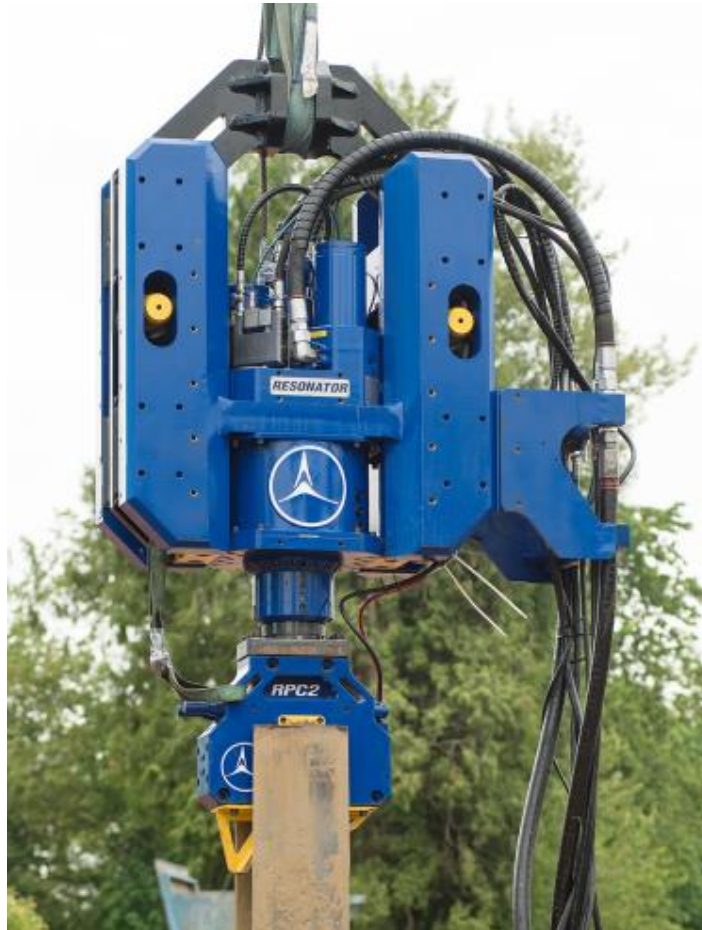
Figure 15-37 Resonant hammer installing an H-pile (courtesy of Resonance Technology).
