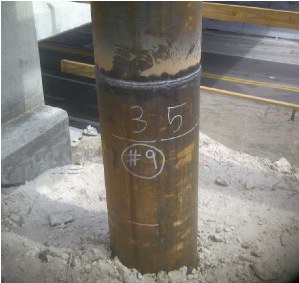
Figure 16-20 Welded pipe pile sections.
