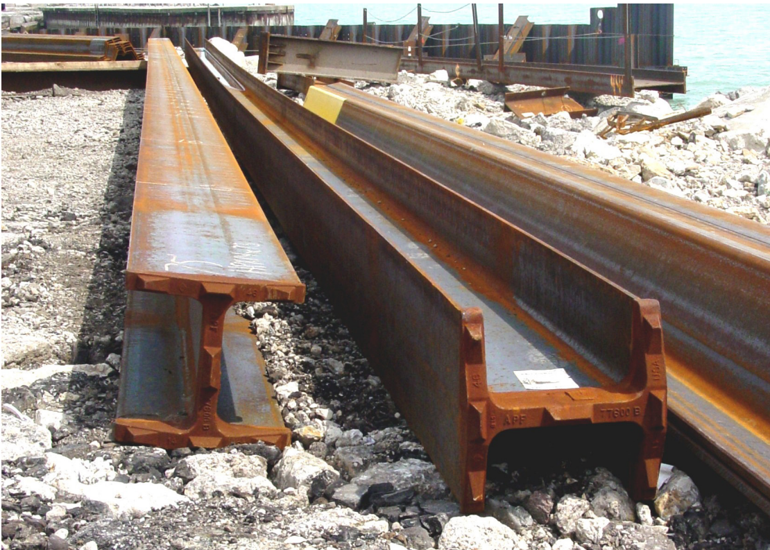
Figure 6-10 H-piles with driving shoes.
