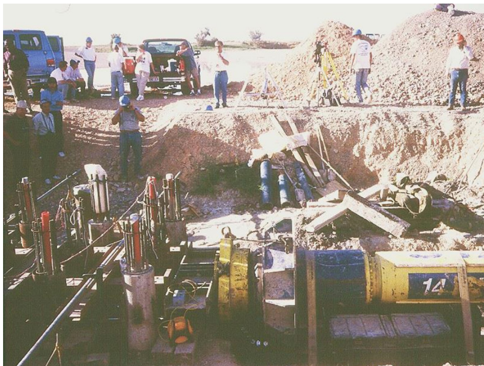
Figure 11-14 Lateral Statnamic test on nine pile group (courtesy of Utah State University).
