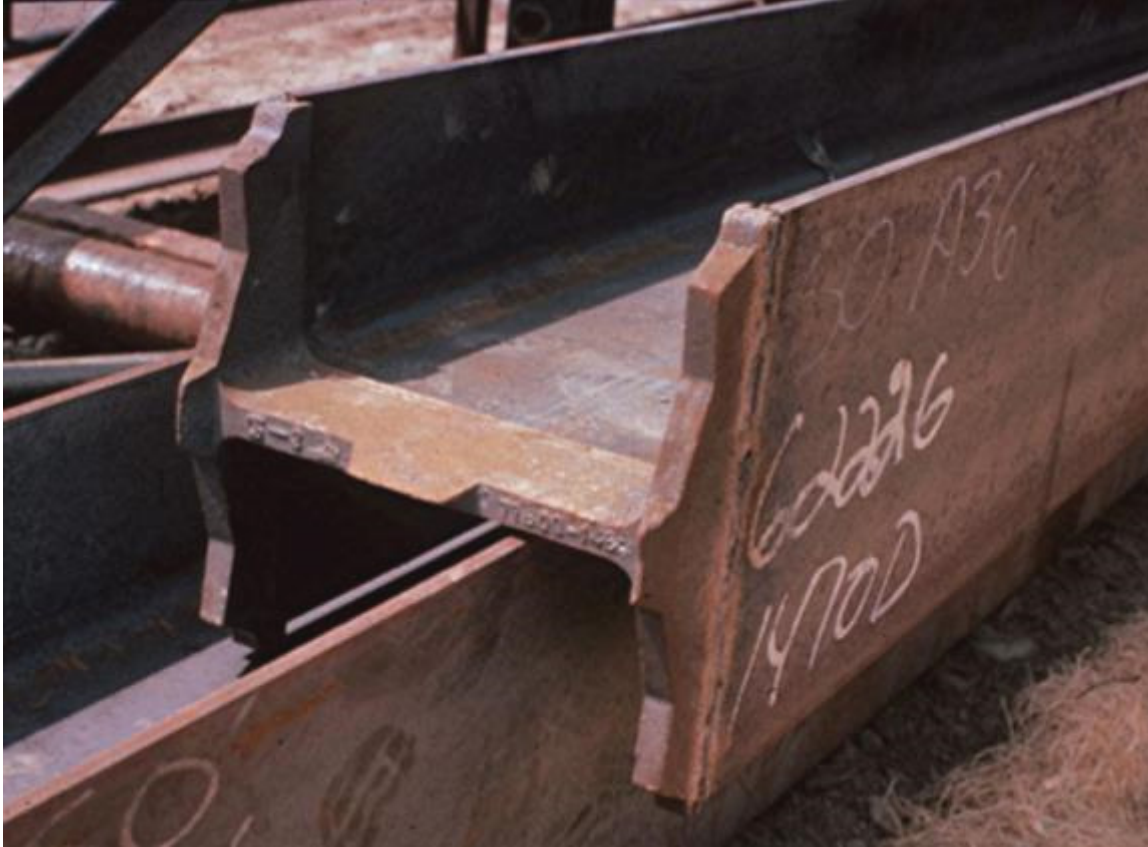
Figure 16-6 Pile shoe welded to pile toe using fillet welds along exterior flanges.
