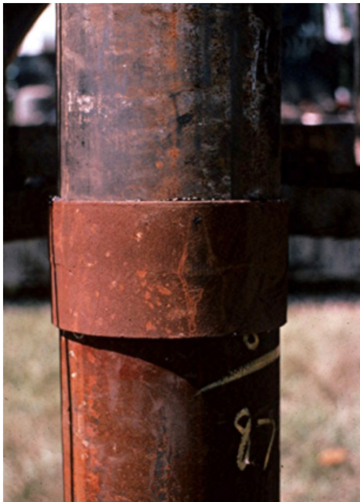
Figure 16-22 Drive-fit mechanical friction splicer on pipe pile.
