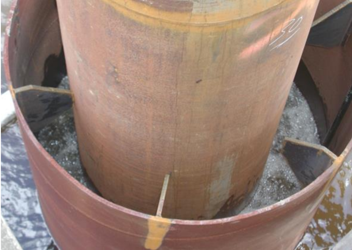
Figure 15-44 Bubble ring with containment device (courtesy of WSDOT).
