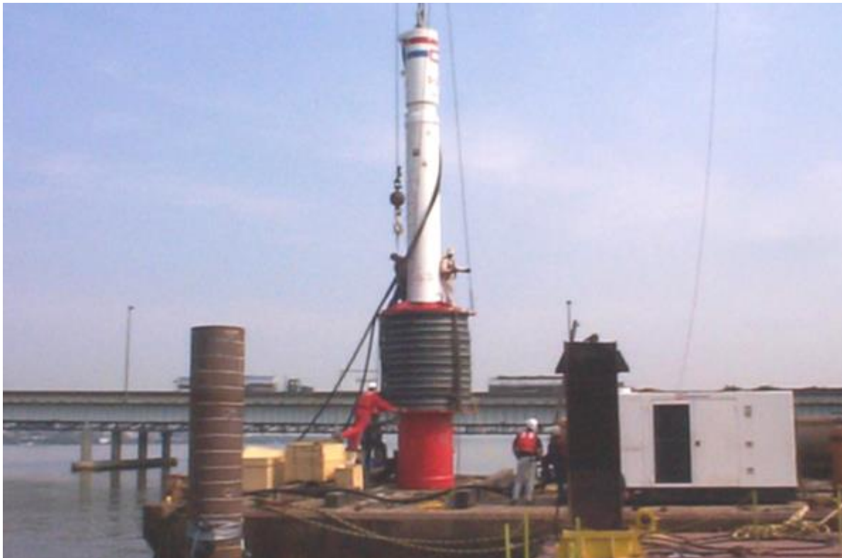
Figure 15-43 Noise shroud for IHC hydraulic hammer.
