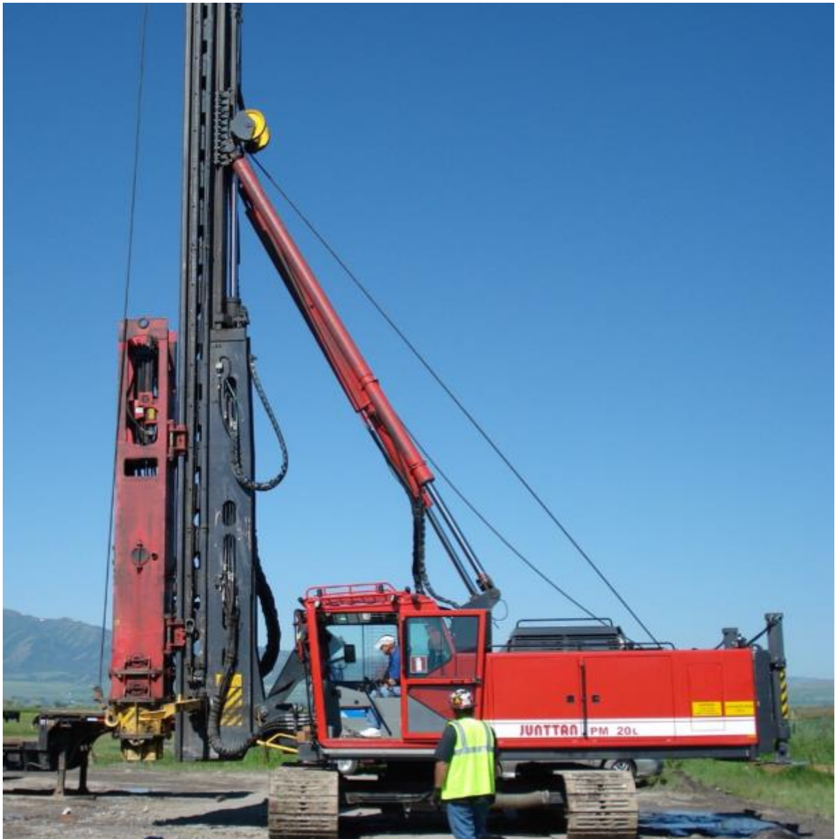
Figure 15-4 Dedicated pile driving system.
