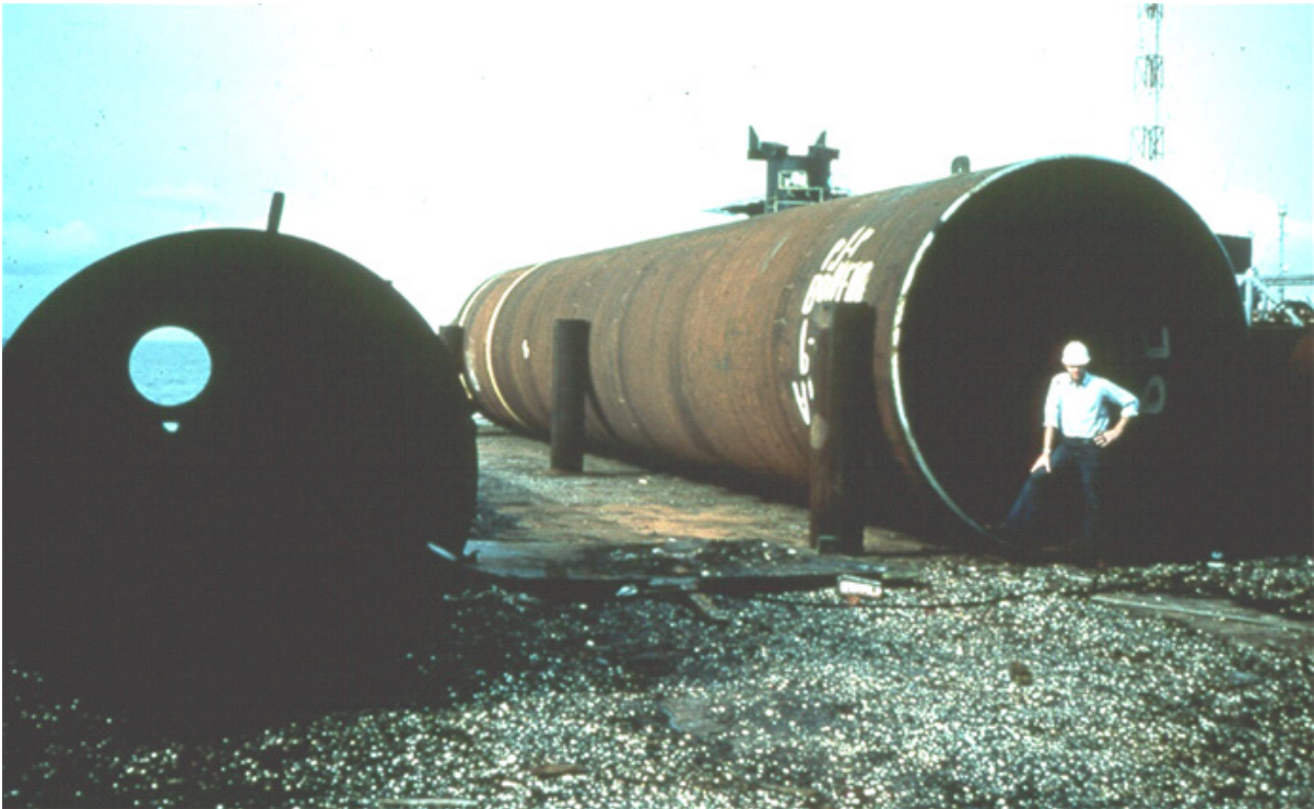
Figure 6-13 Large diameter open end pipe piles.
