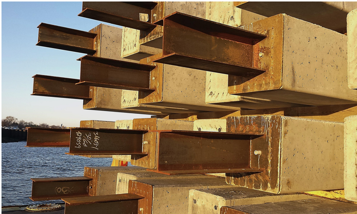
Figure 6-24 Precast concrete piles each with H-pile stinger.
