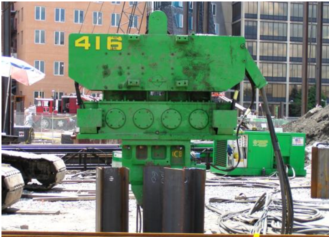
Figure 15-36 Vibratory hammer installing an H-pile (courtesy ICE).
