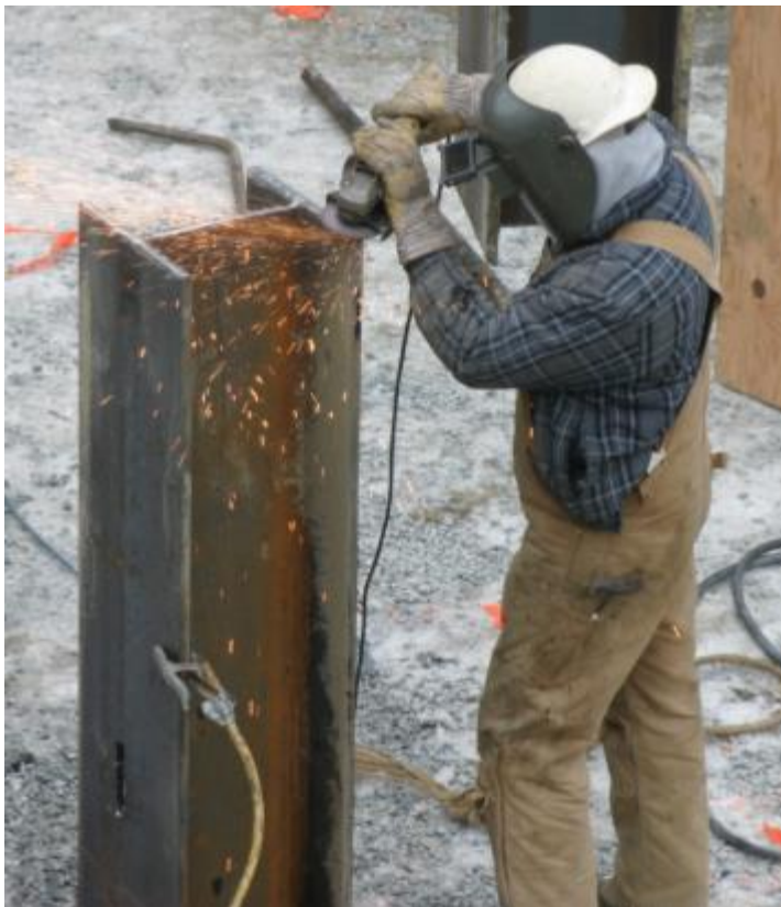
Figure 16-37 Grinding edges of web and flange in preparation for weld.
