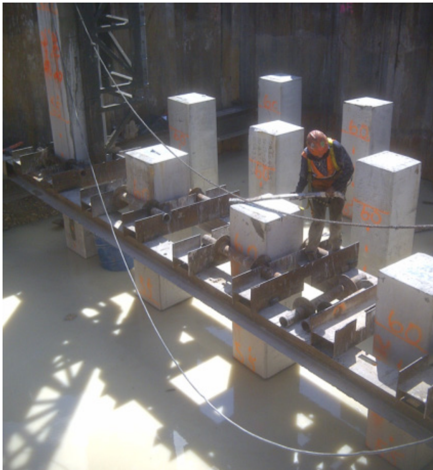
Figure 15-16 Template system.
