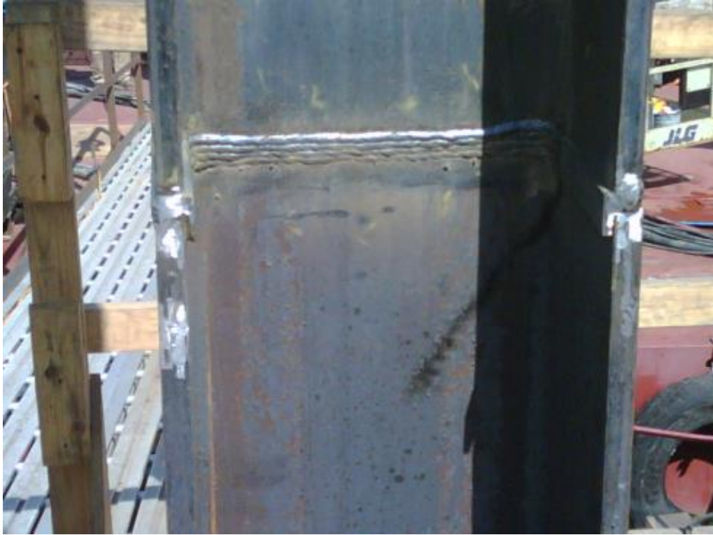
Figure 16-7 Full penetration groove weld with backer bars.
