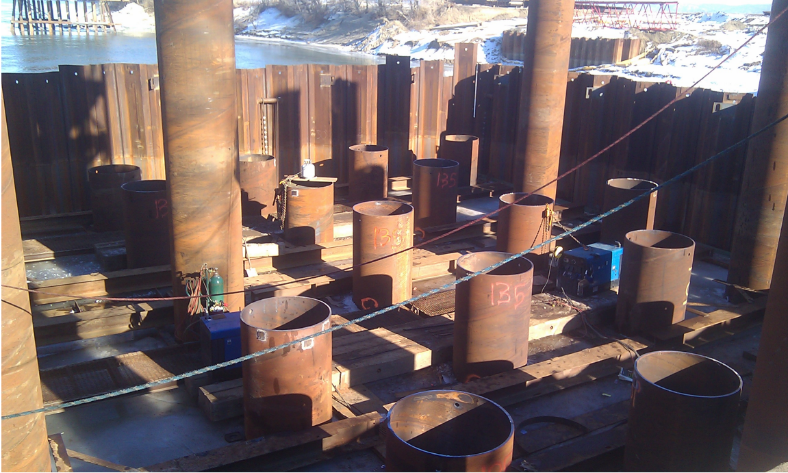
Figure 6-12 42 inch diameter, spiral weld, open end, pipe for main river pier.
