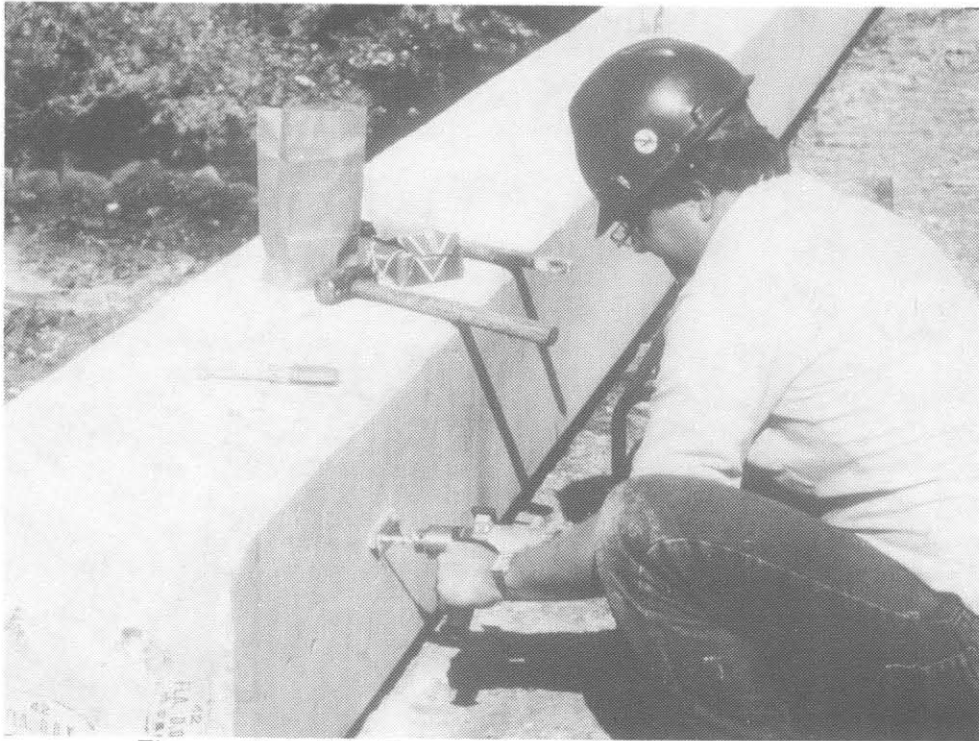
Figure 18.1 Pile Preparation for Dynamic Testing
