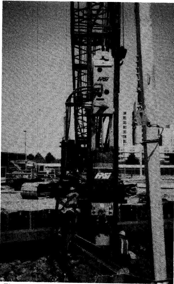
Figure 22.23 Single Acting Hydraulic Hammer
