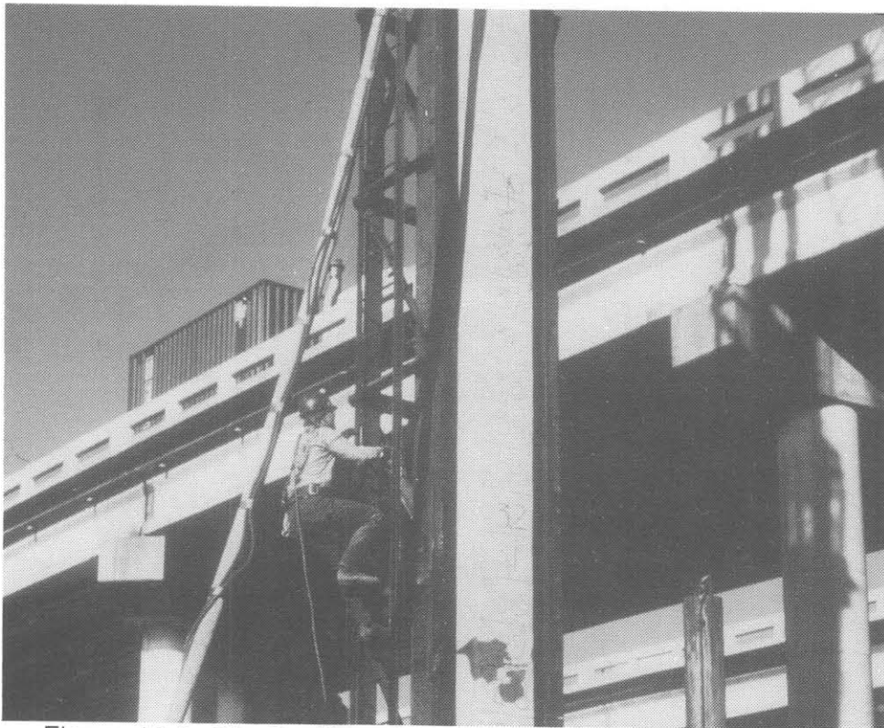
Figure 18.2 Pile Positioned for Driving and Gage Attachment
