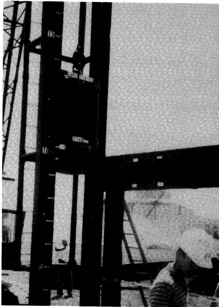
Figure 22.12 Typical Drop Hammer
