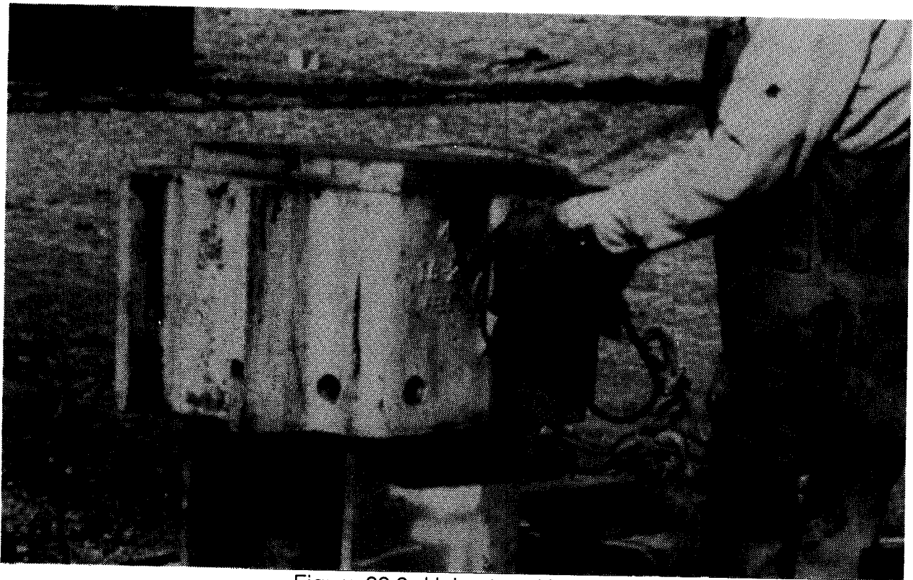
Figure 22.9 Helmet on H-pile
