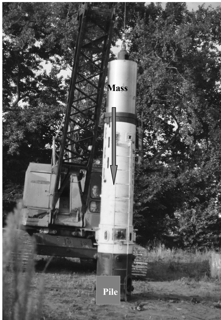
Figure I-6 : Dynamic loading test (crane + mass + pile)
