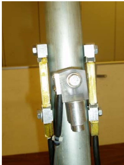
Figure 8-6 Installation of strain gages and accelerometers
